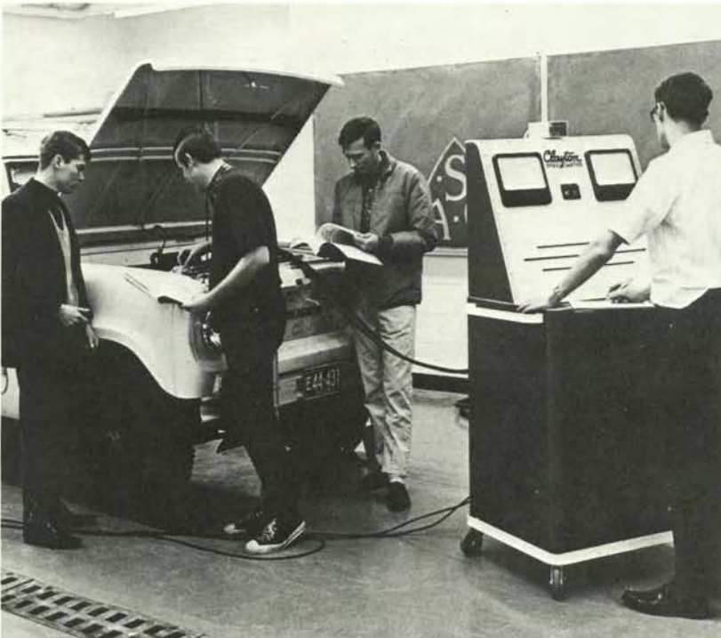
Students measure automotive emissions for exhaust-air pollution study.
