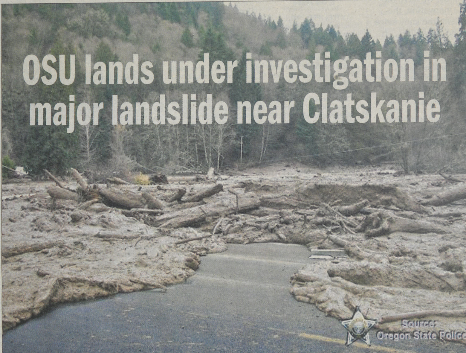
PHOTO COURTESY THE OREGON STATE POLICE The cause of the massive landslide over winter break on US Highway 30 near Clatskanie, Ore. is being investigated, and has yet to be determined.
