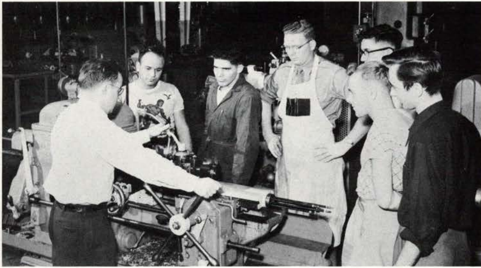
Keith Soderlund demonstrates a metal lathe during an industrial arts class.
