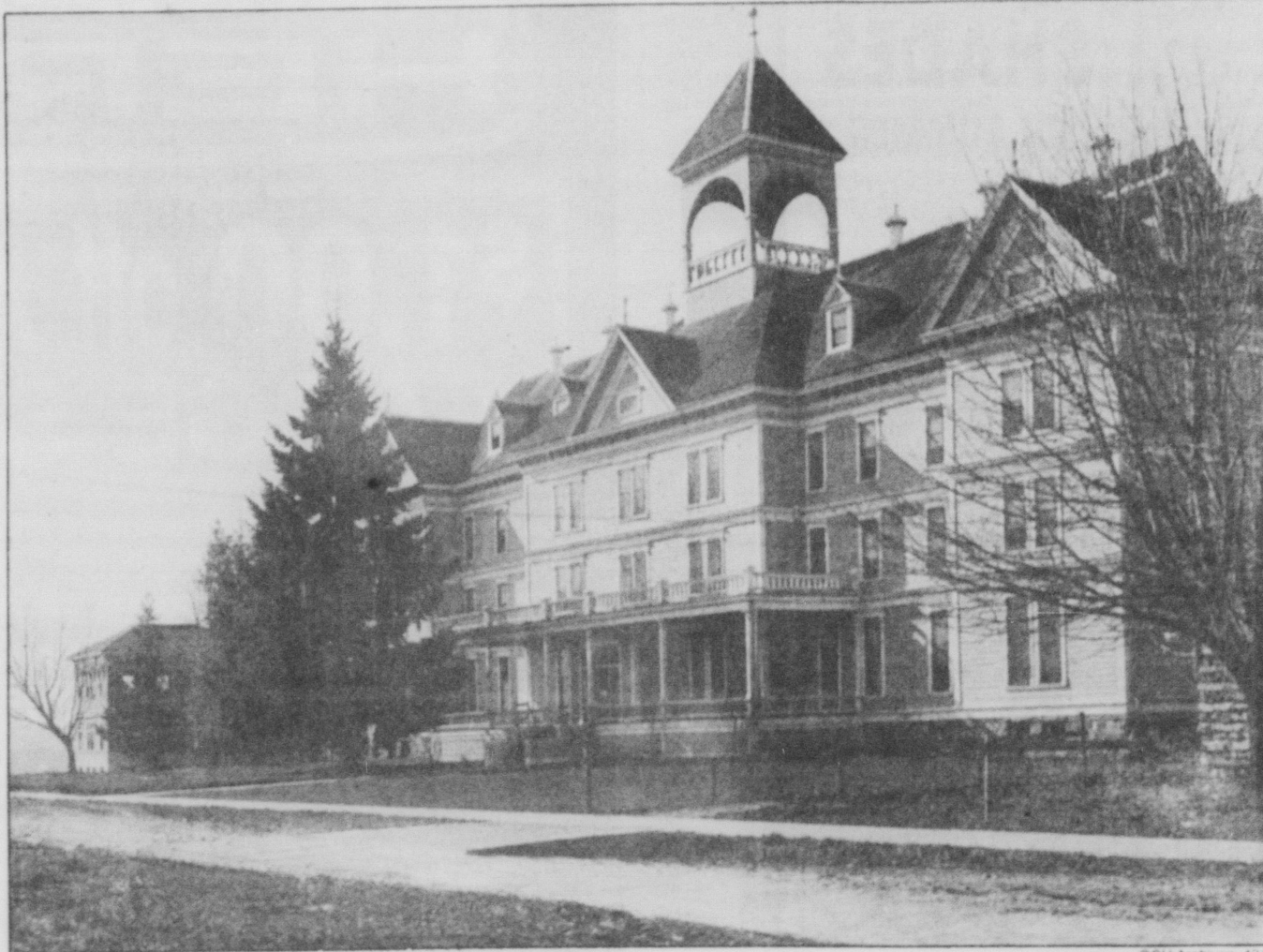
Fairbanks Hall, which was constructed in 1872 under the name of Cauthorn Hall, has also borne the name of Kidder Hall at one time or another.
