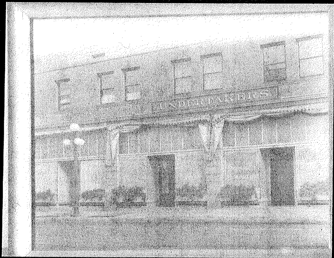
Original store-front at NE Union and Russel
