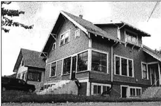
Photo 3: 10th and Maple, facing Northwest
