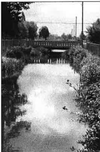
Photo 5: Canal from 11th, facing North
