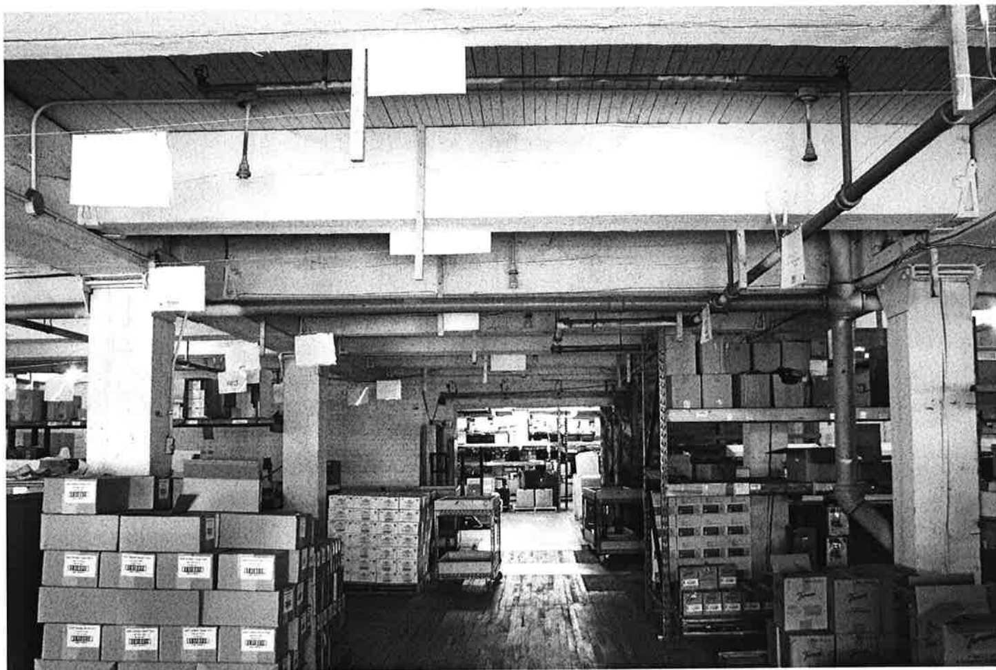
Photo 17 of 23: Second floor: warehouse. View to NW.
