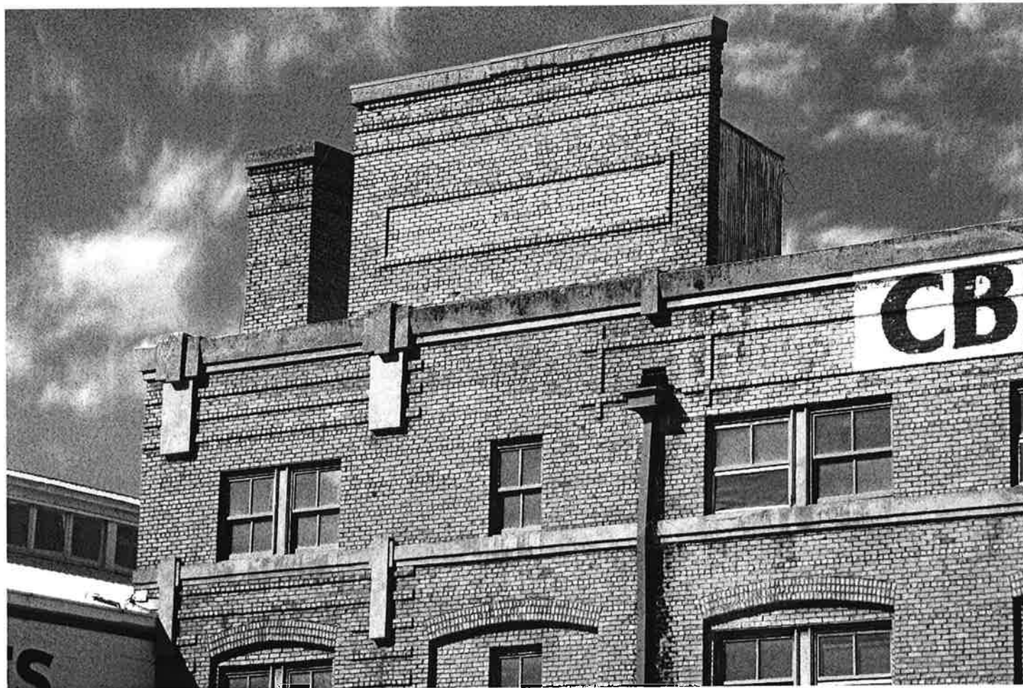
Photo 9 of 23: Southwest façade: parapet, chimney, and elevator overrun detail. View to NE.
