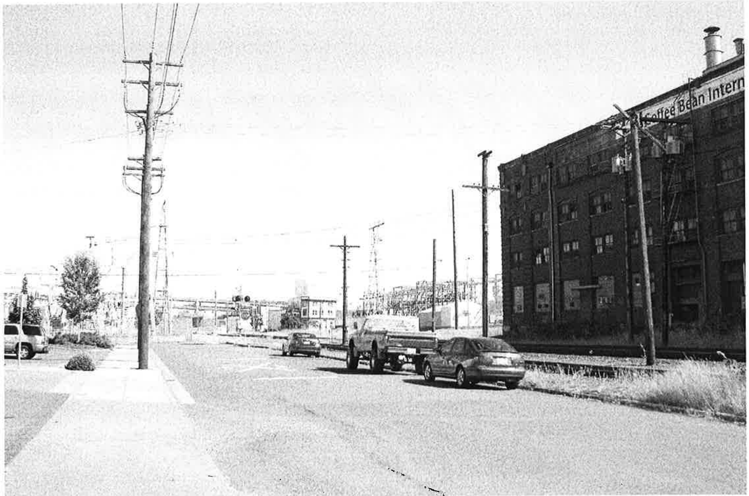
Photo 6 of 23: Northeast façade and surrounding neighborhood. View to NW.
