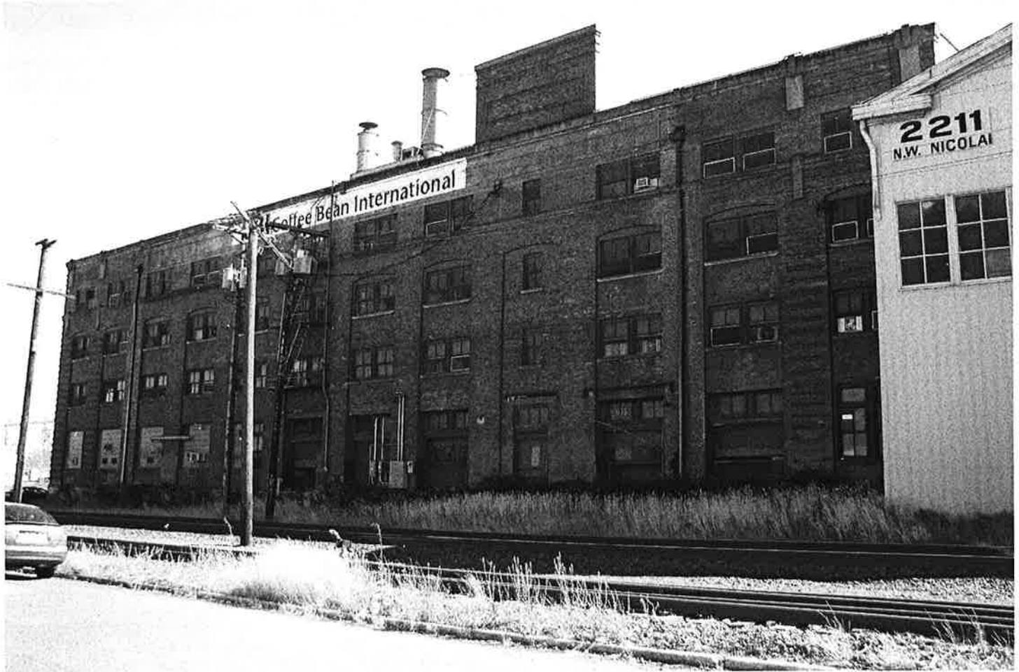
Photo 5 of 23: Northeast façade. View to NW.
