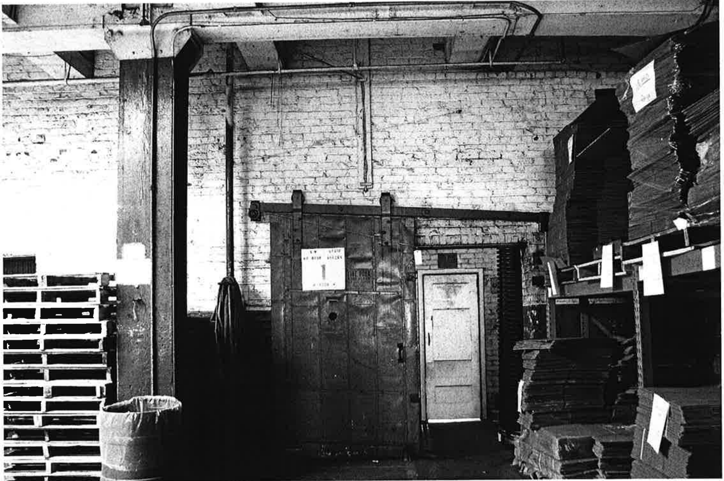
Photo 16 of 23: First floor: warehouse fire door. View to SE.
