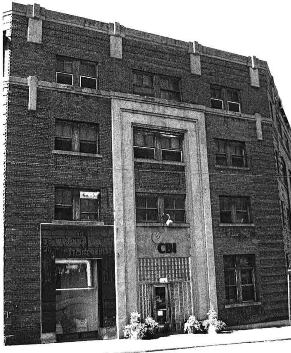
Photo 1of 23: Entry/south façade. View to N.
