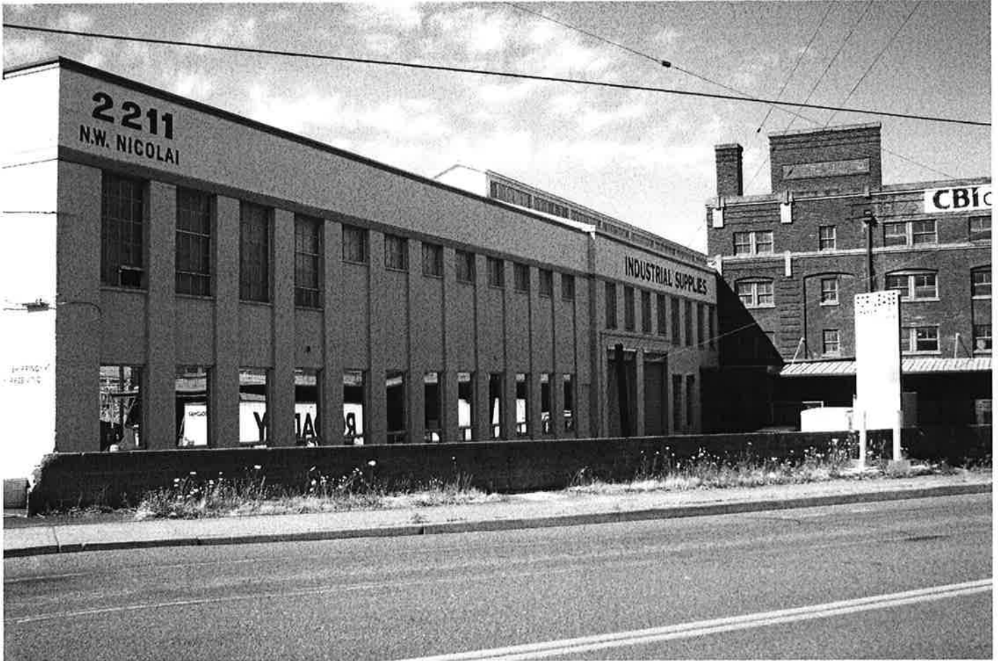
Photo 7 of 23: Southwest façade and adjacent building. View to N.
