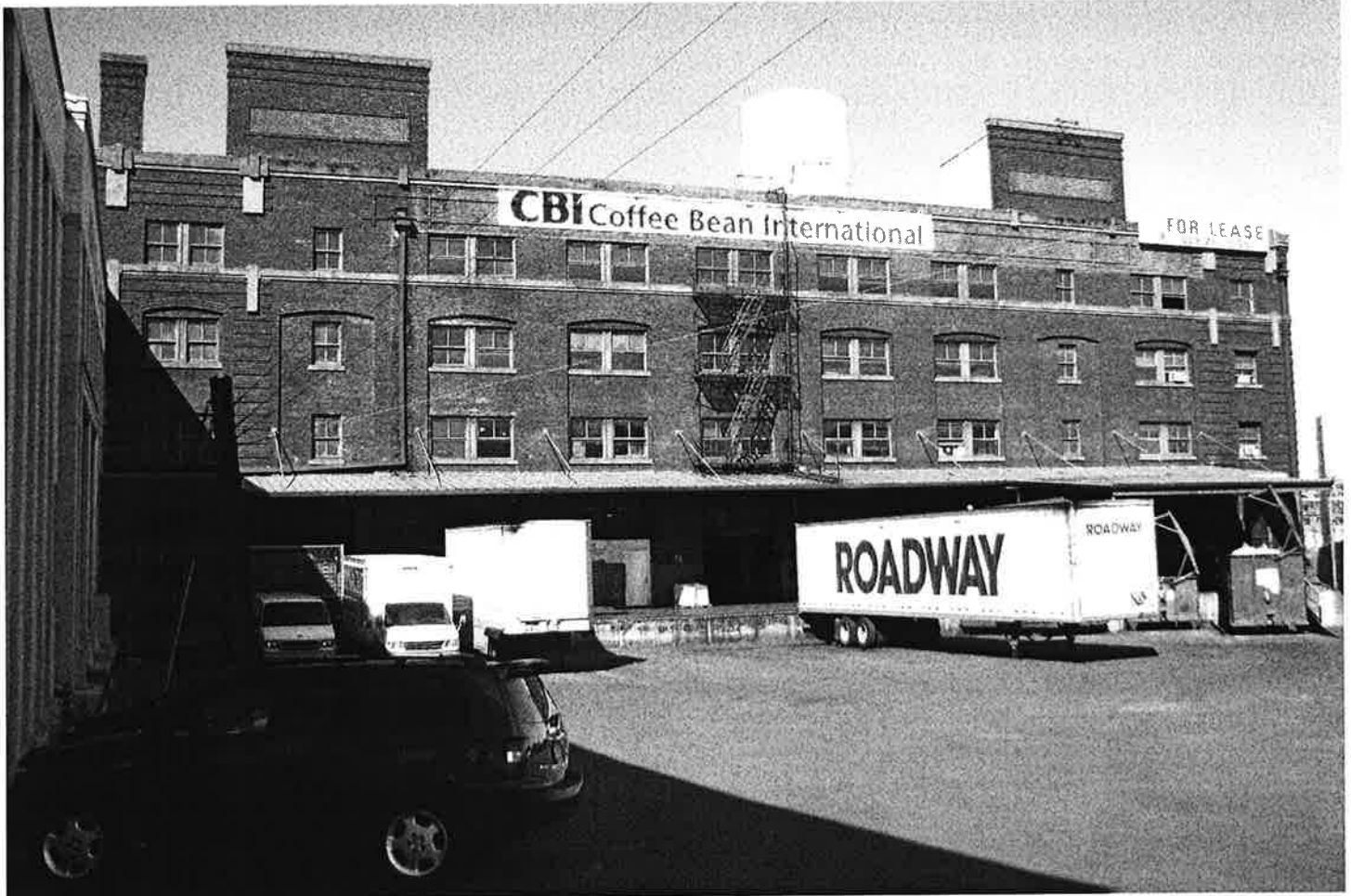
Photo 4 of 23: Southwest façade. View to NE.
