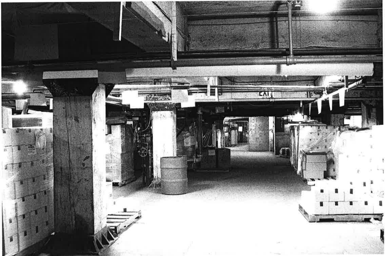
Photo 21 of 23: Basement: warehouse. View to SW
