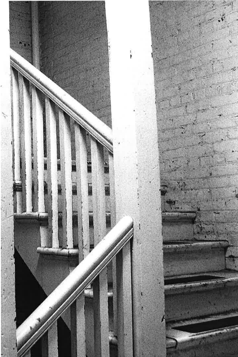
Photo 23 of 23: Warehouse stair.
