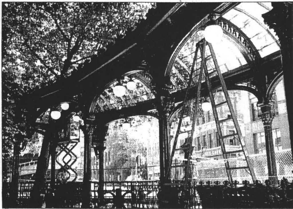
Heidi Seidelhuber, contractor for rebuilding the Pioneer Square pergola, called the accident that took down the 1909 structure "a blessing in disguise." Photo by Sam Bennett
