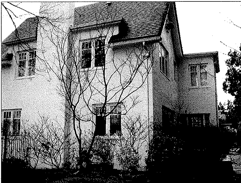
4 of 16: Exterior view of the Northwesterly elevation at the rear looking east at the westerly wing
