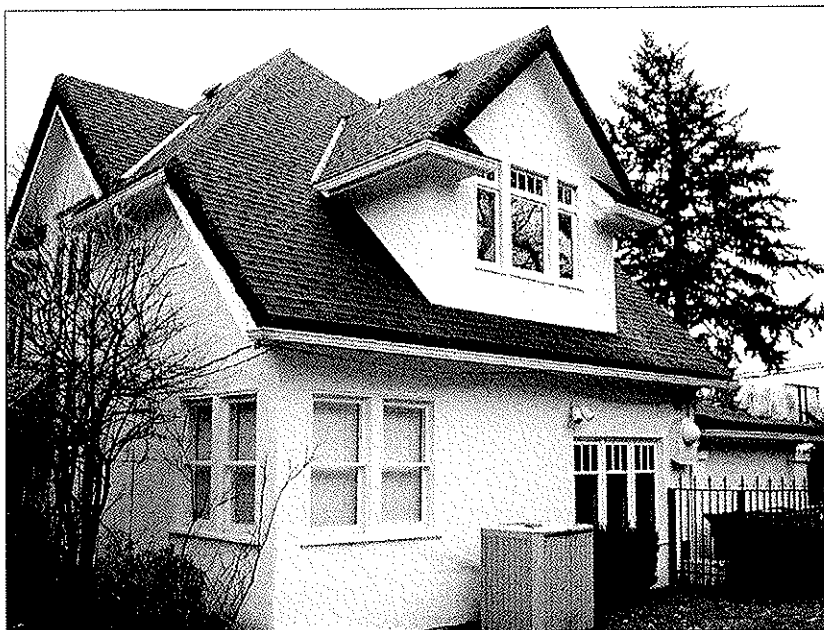
6 of 16: Exterior view of the Southwesterly and southeasterly elevations looking westerly
