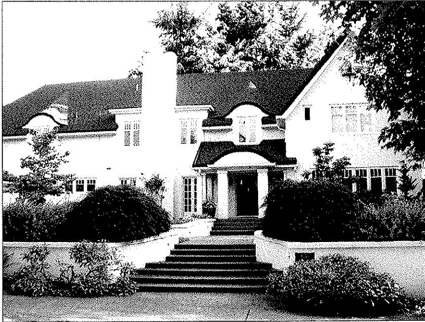
1 of 16: Exterior view of Northeast elevation looking southwest
