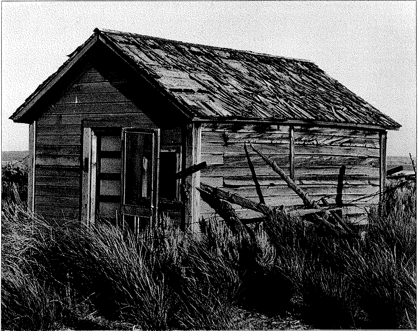
6 of 31: Exterior: Bunkhouse #1, south and east facades, facing northwest, 2004
