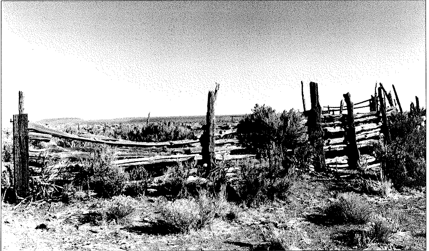
17 of 31: Exterior: Fencing, facing east, 2007
