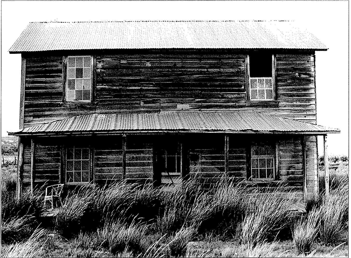
2 of 31: Exterior: Ranch house, south façade (front), facing north, 2004
