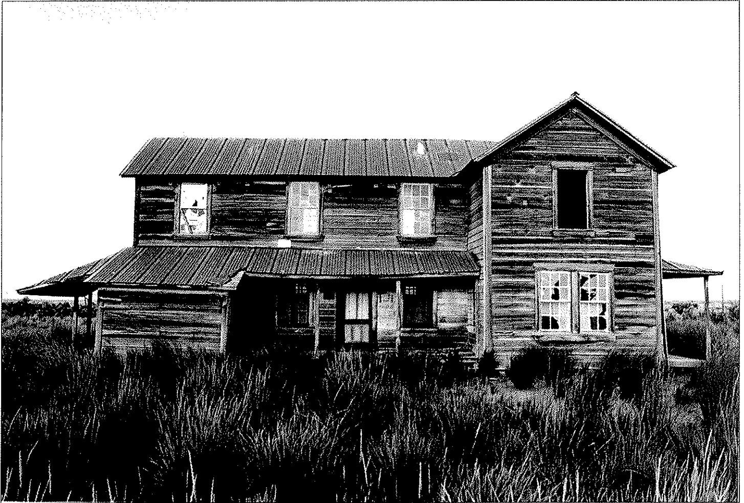
5 of 31: Exterior: Ranch house, west façade, facing east, 2004
