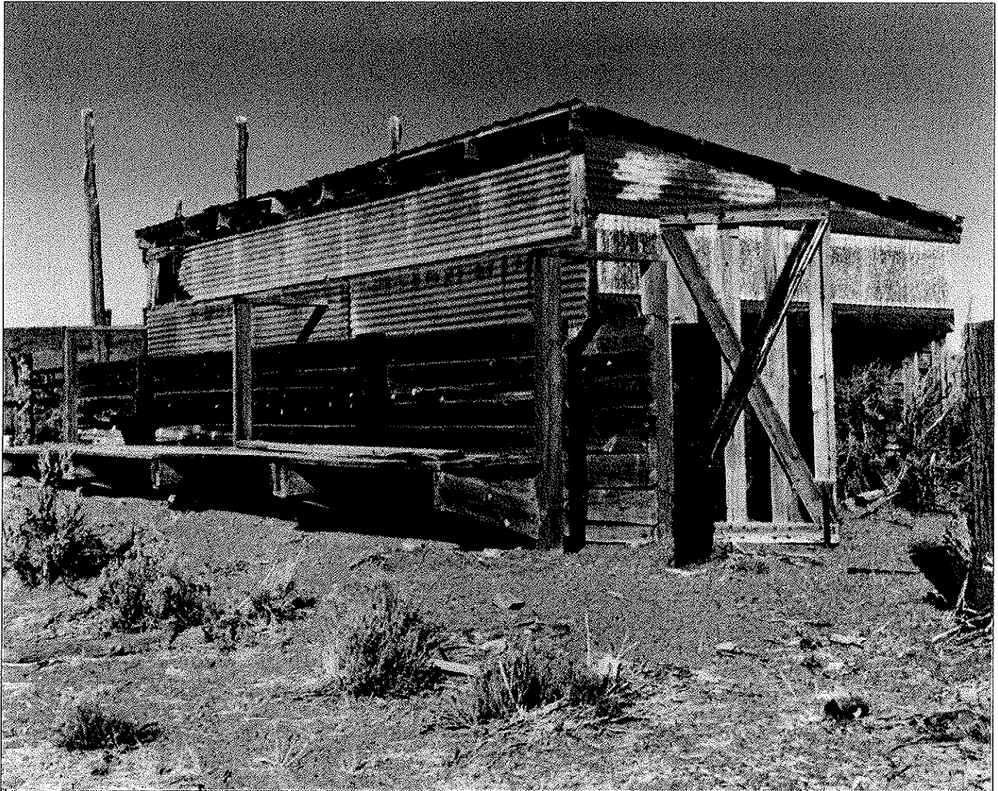
19 of 31: Exterior: Animal paddock, south and west facades, facing northeast, 2007
