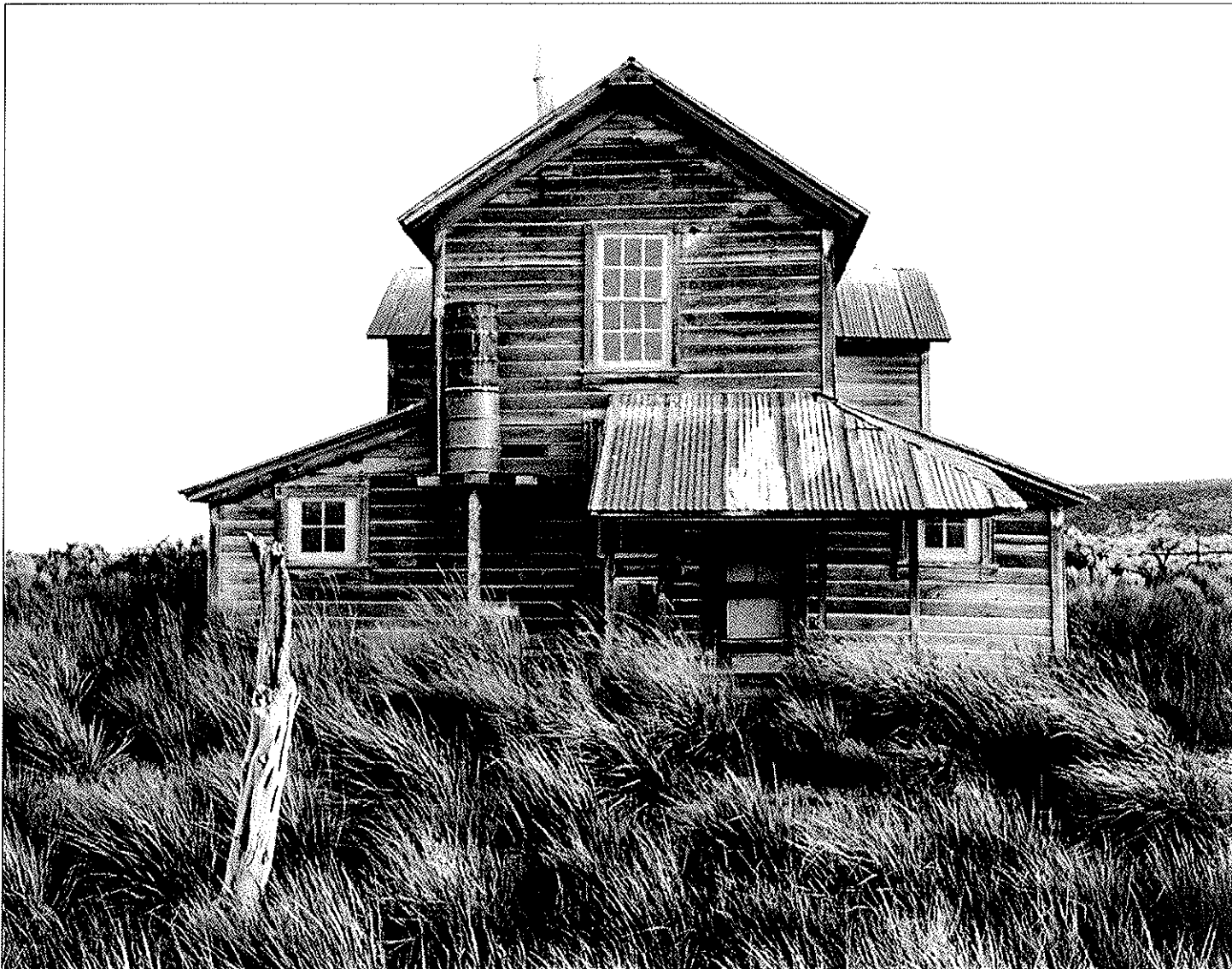
3 of 31: Exterior: Ranch house, north façade (back), facing south, 2004
