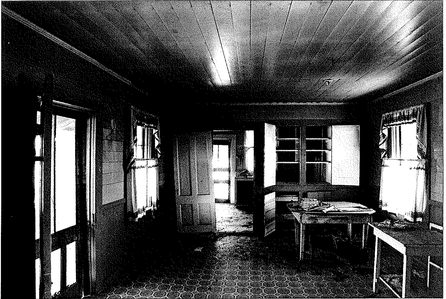
27 of 31: Interior Main Ranch House: Living room, facing north, 2004
