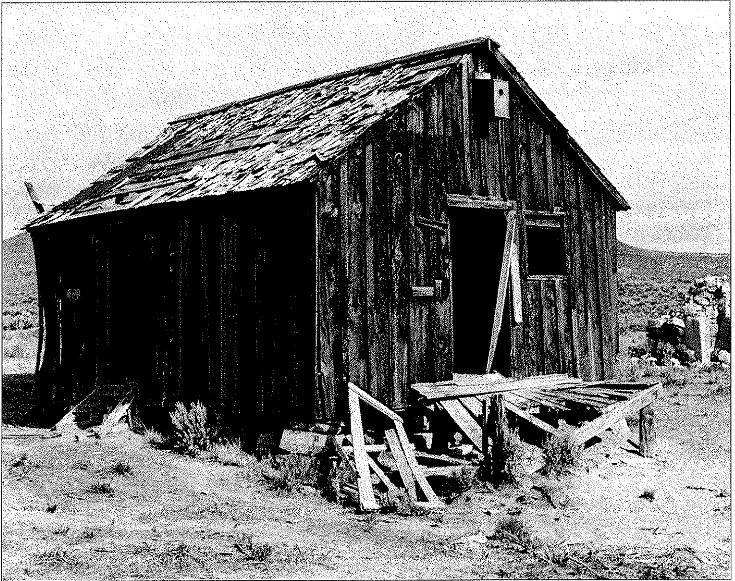
7 of 31: Exterior: Bunkhouse #2, south and east facades, facing northwest, 2004
