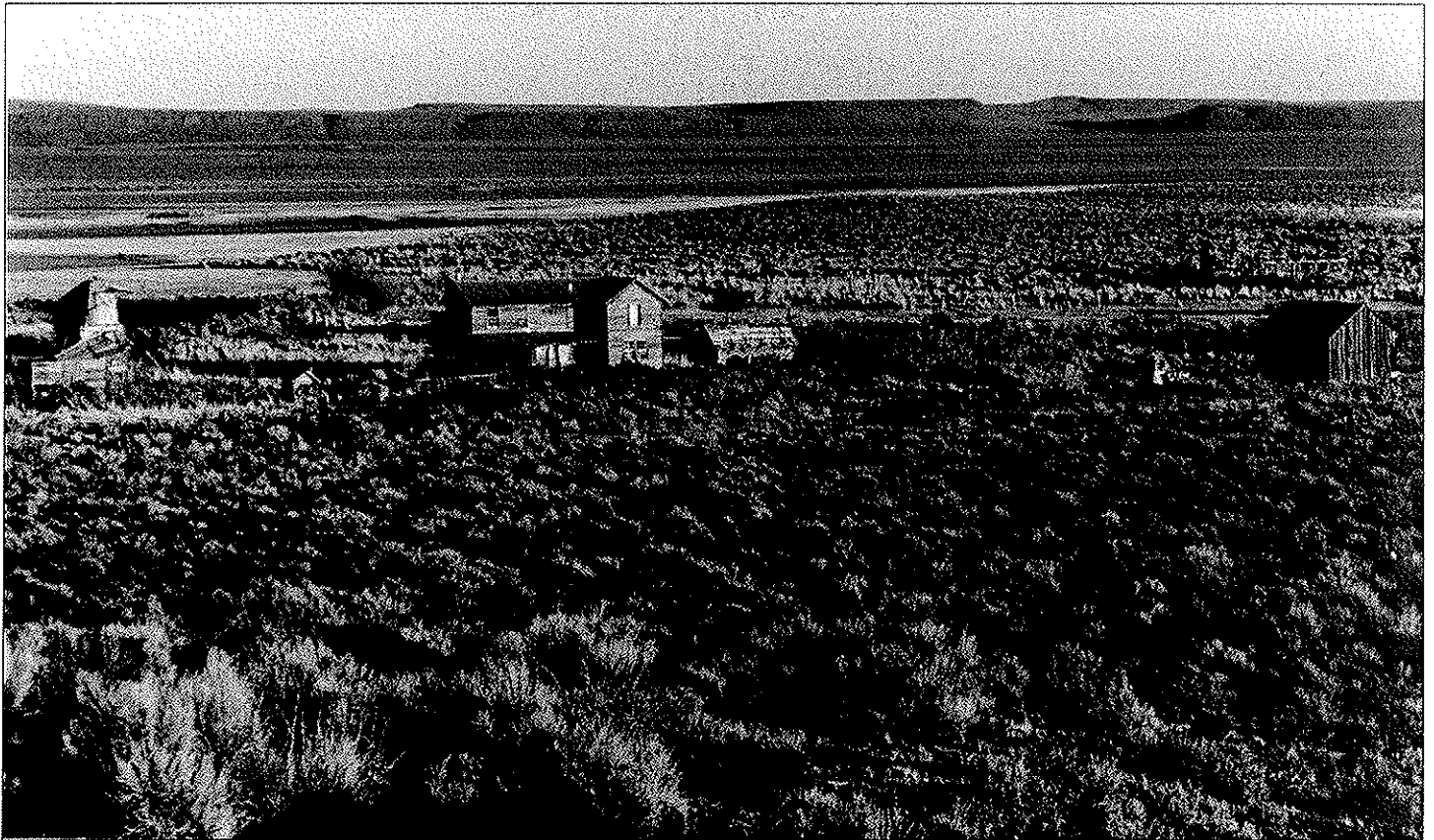
1 of 31: Exterior: Overview of Shirk Ranch, facing southeast, 2007
