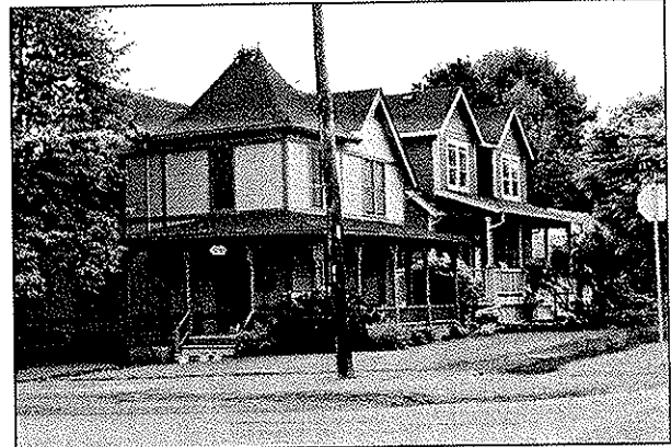
20 of 21: 6 th Ave, facing SW
