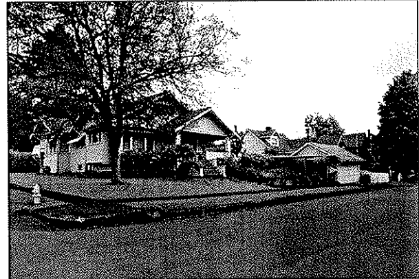
8 of 21: 13 th St and 4 th Ave, facing NE
