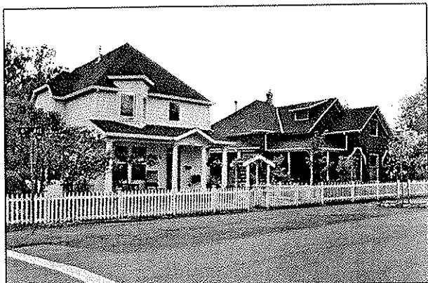
17 of 21: 12 th St and 6 th Ave, facing SW
