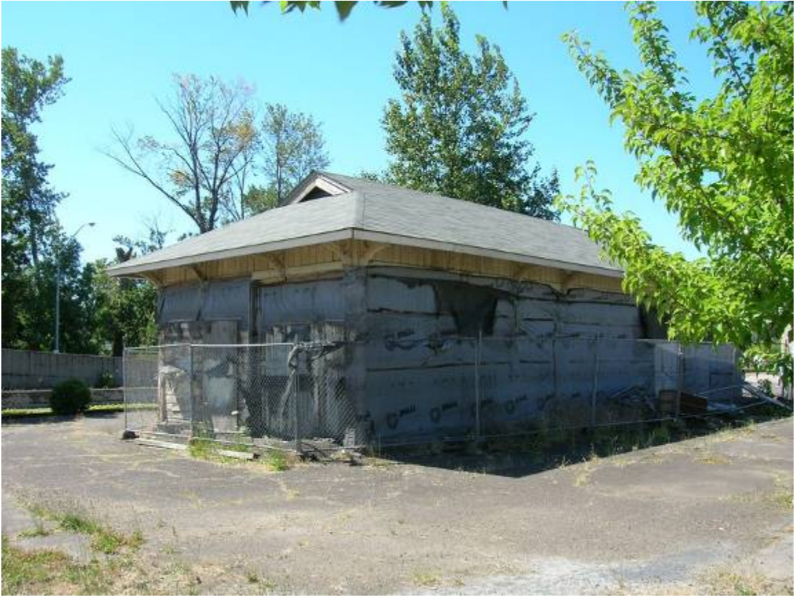
9 of 11. REA Depot, Northwest Elevations
