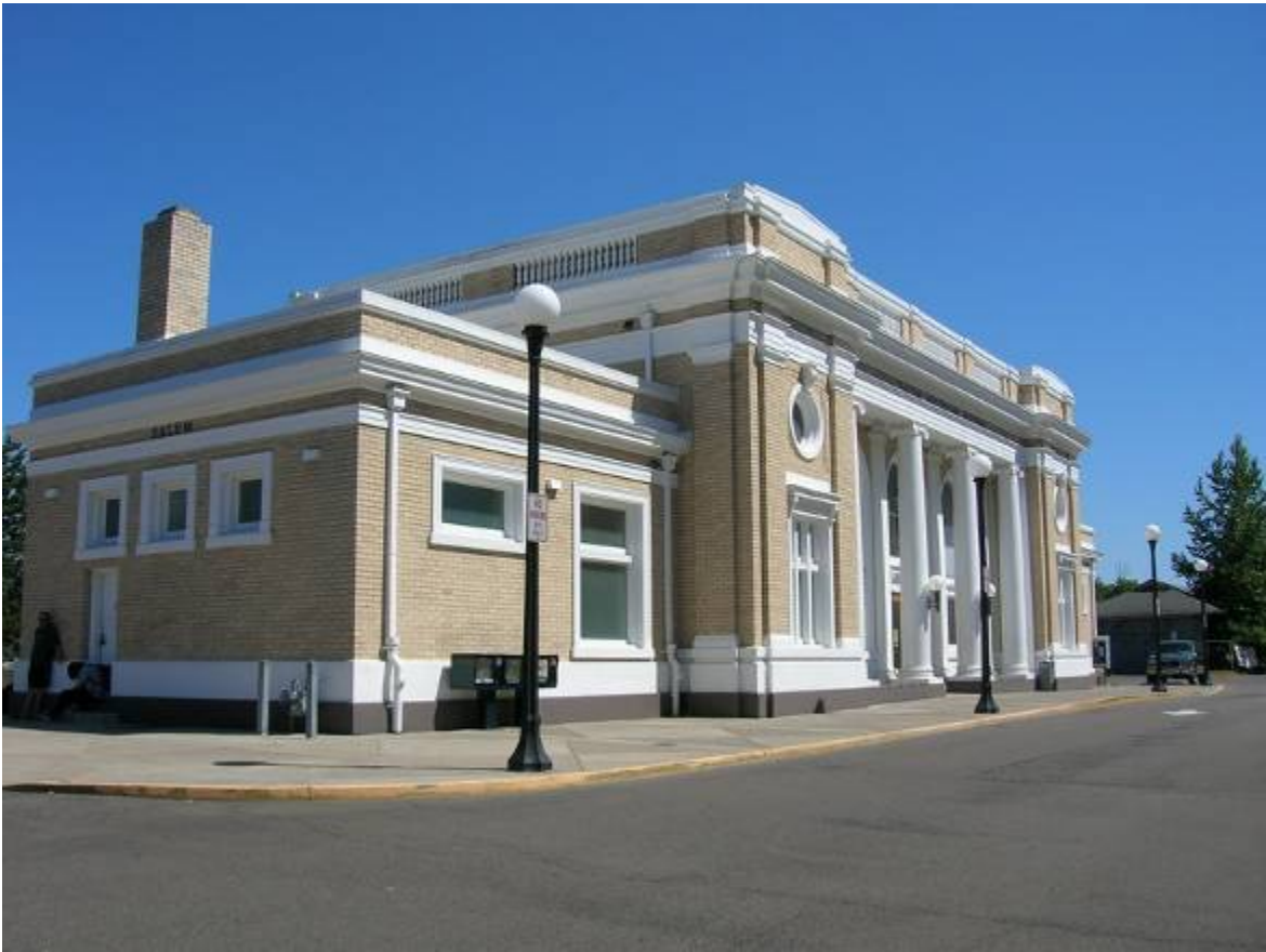
1 of 11. Salem Southern Pacific Railroad Depot, West Elevation
