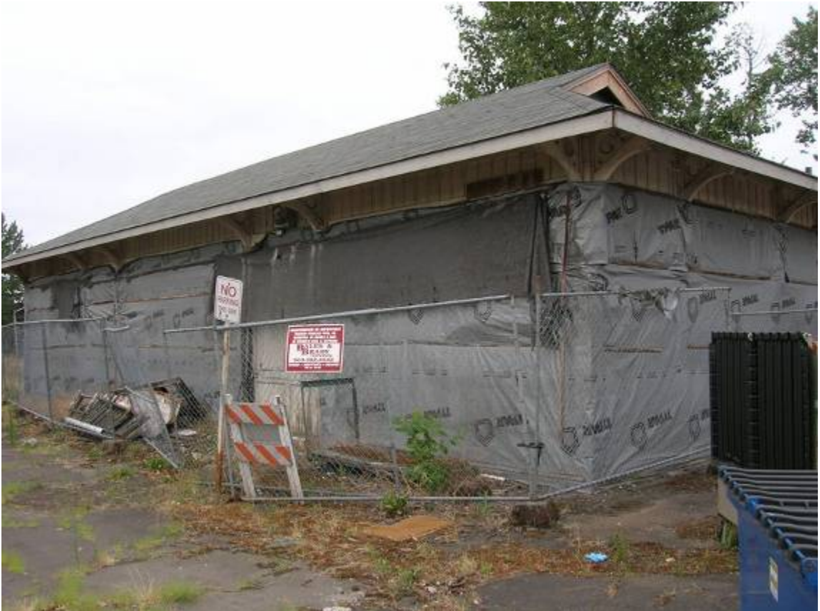
10 of 11. REA Depot, Northwest Elevation
