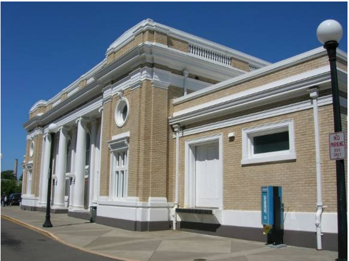
2 of 11. Salem Southern Pacific Railroad Depot , West Elevation
