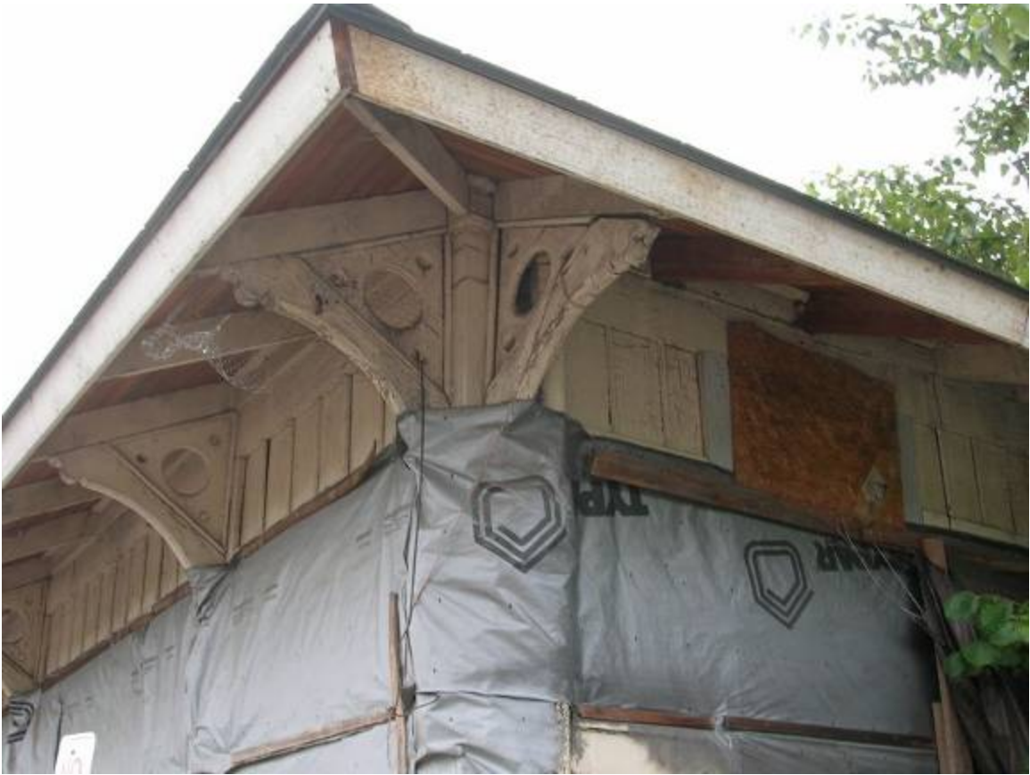
11 of 11. REA Depot, Detail of roof brackets
