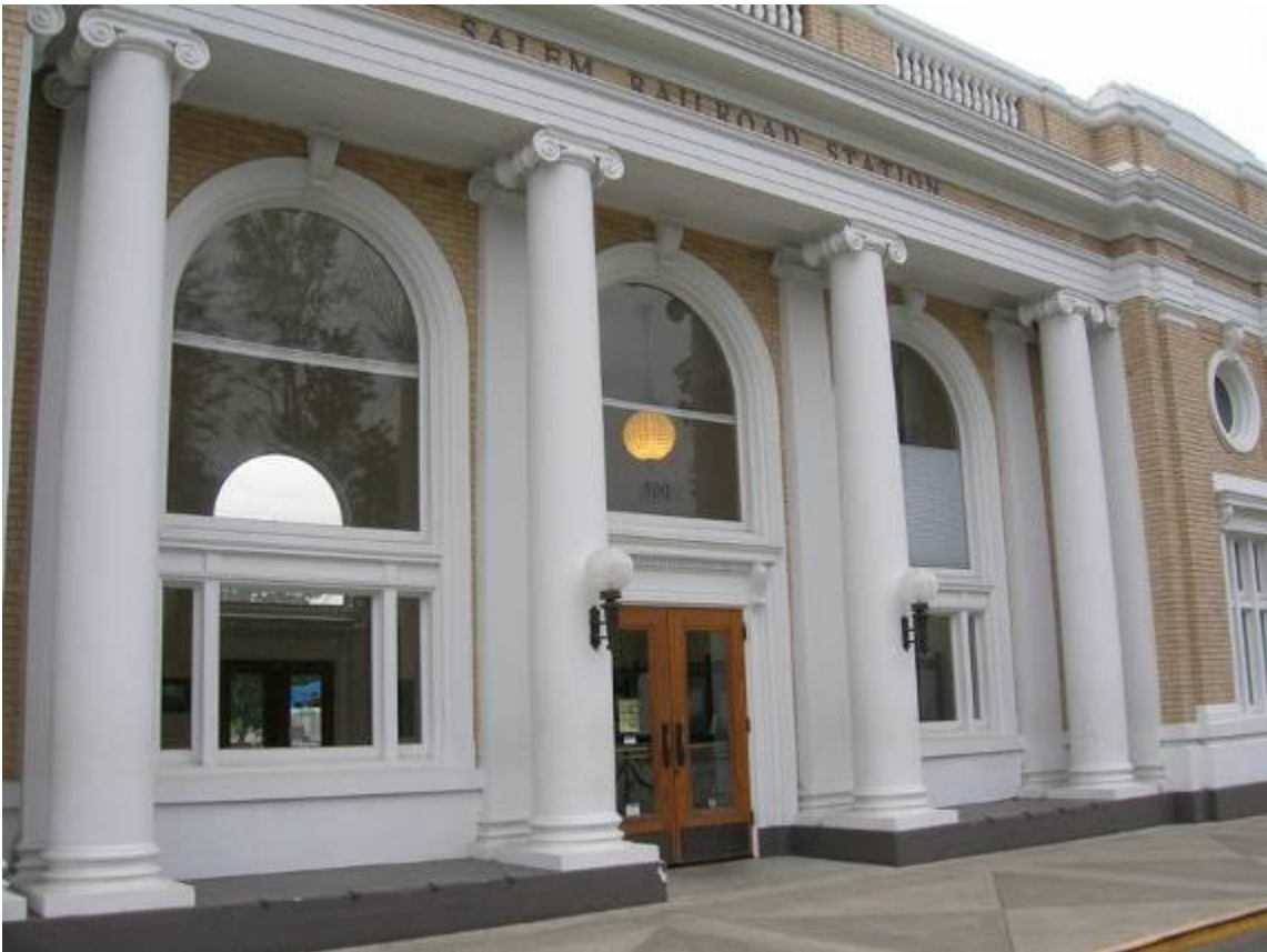
4 of 11. Salem Southern Pacific Railroad Depot , West Elevation
