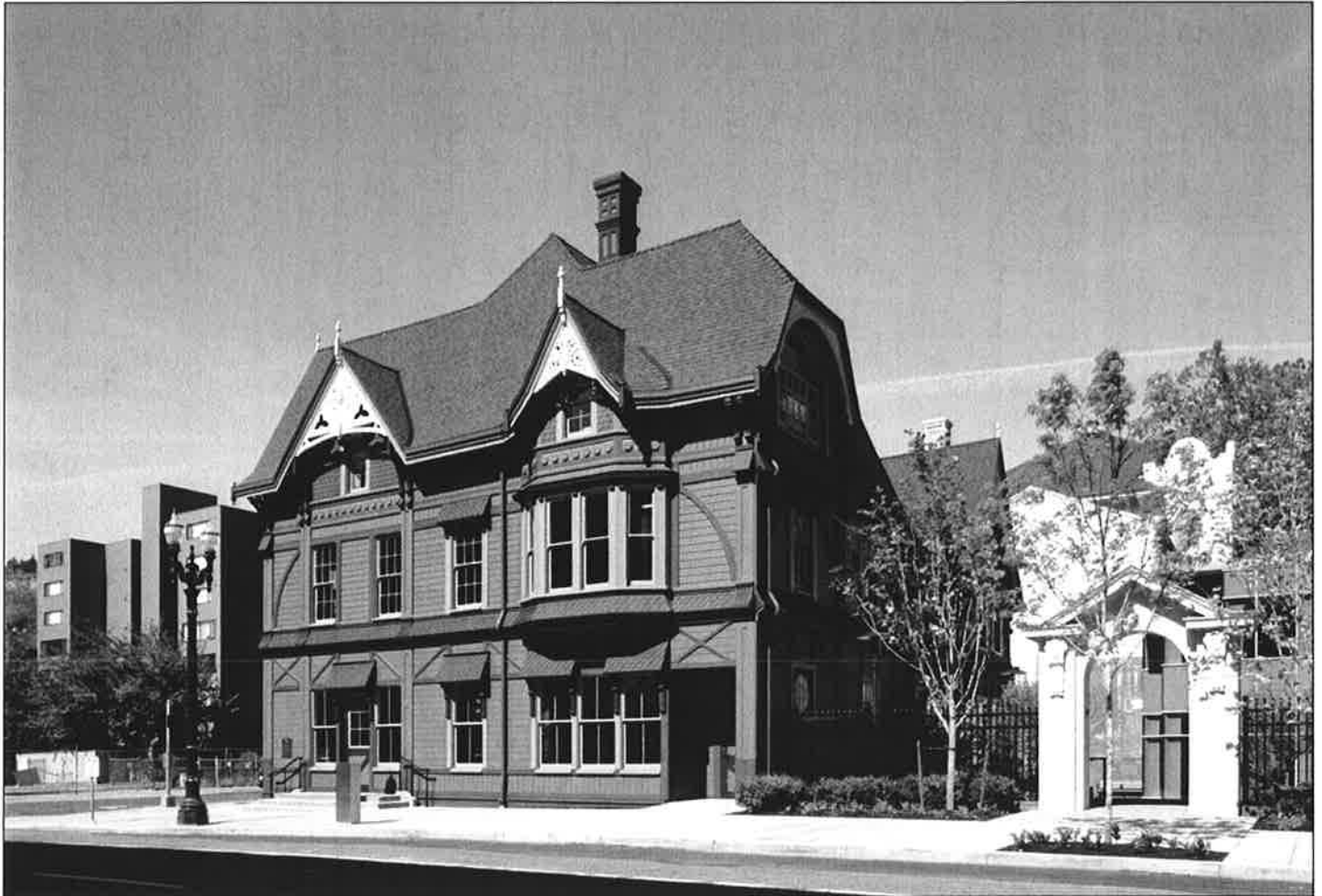
1 of 15: East facade. View to W.
