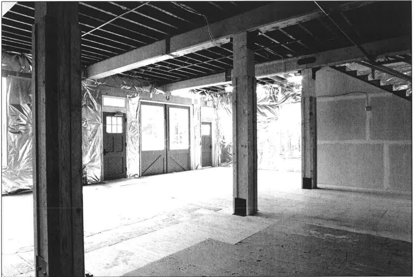
11 of 15: First floor. View to SW.
