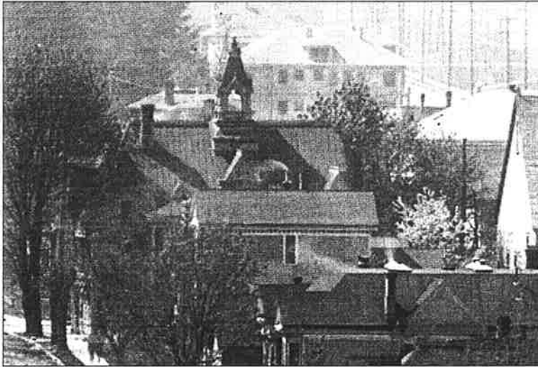
Image 4. 1908 photograph showing Ladd Carriage House from the north. Source: Oregon Historical Society, OrHi 67367.
