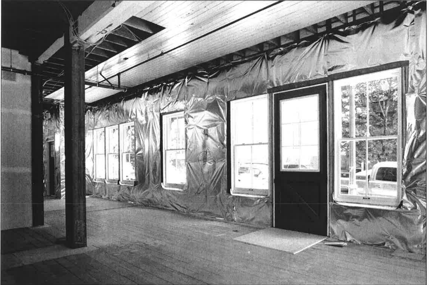
9 of 15: First floor: SW Broadway entrance. View to NE.
