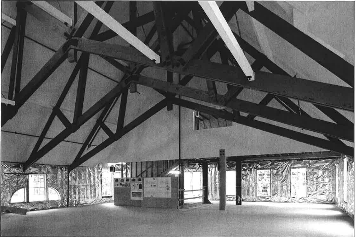
14 of 15: Second floor. View to E.
