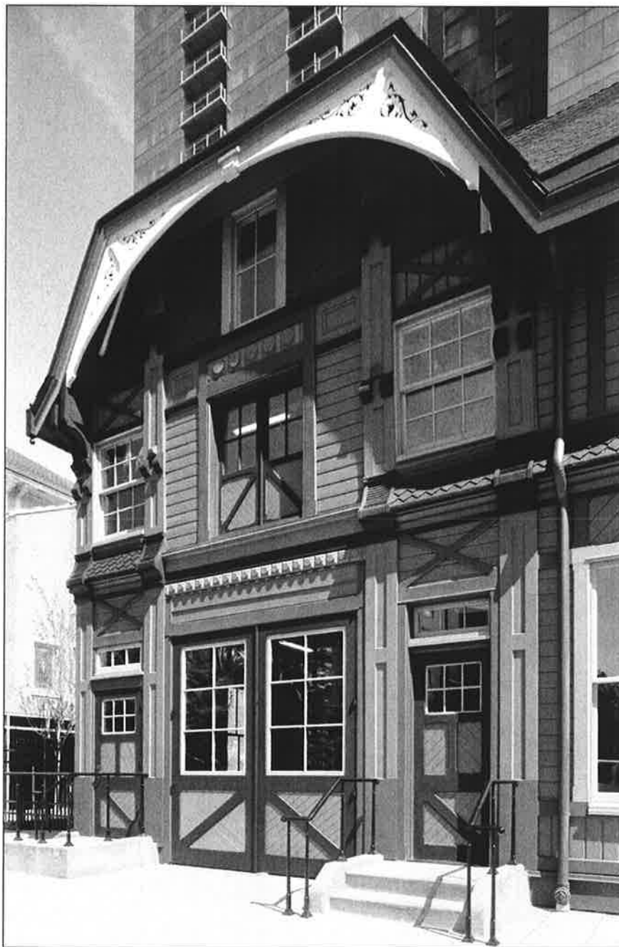
5 of 15: South façade: detail of eastern-most bays. View to N.
