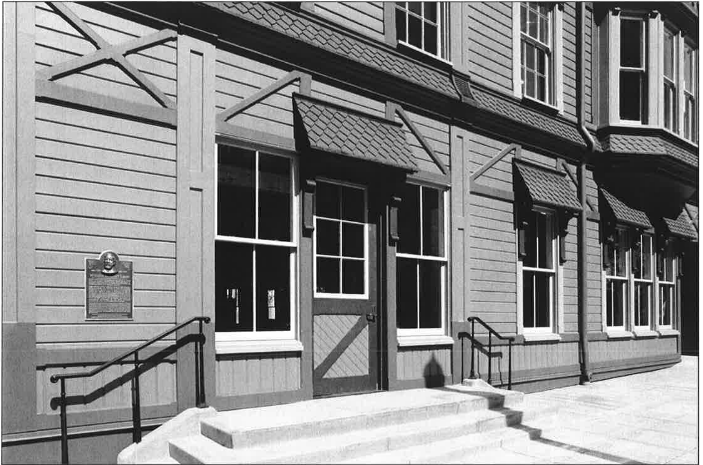
3 of 15: East façade: detail of ground floor. View to NW.
