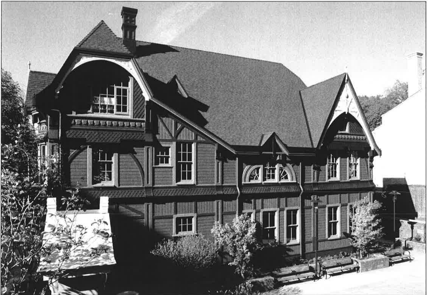
7 of 15: North façade. View to SW.
