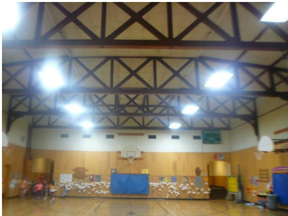
Gymnasium facing north
