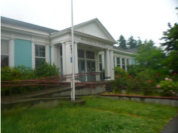
East elevation facing northwest
