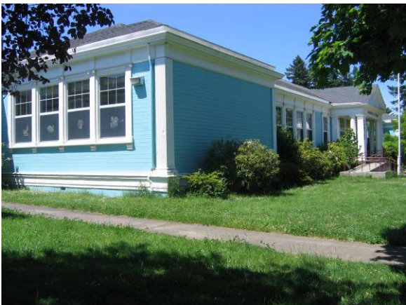
Column detail facing southwest
