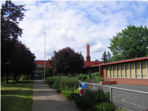
Entry courtyard with south and west elevations
