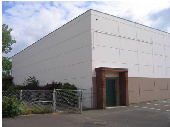
North elevation facing southeast
