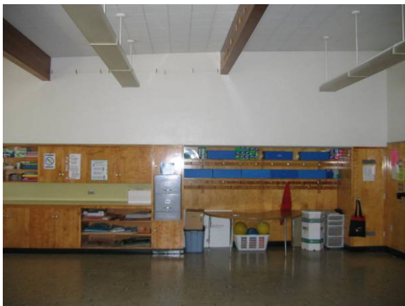
Classroom built-ins, beams and ceiling
