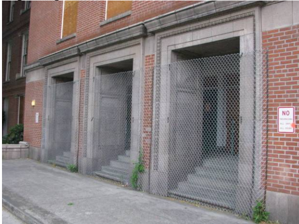
Main building (370A), detail of front portal entrances, looking northeast.
