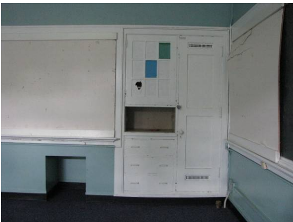
Main Building (370A), representative built-in cabinets in classroom.
