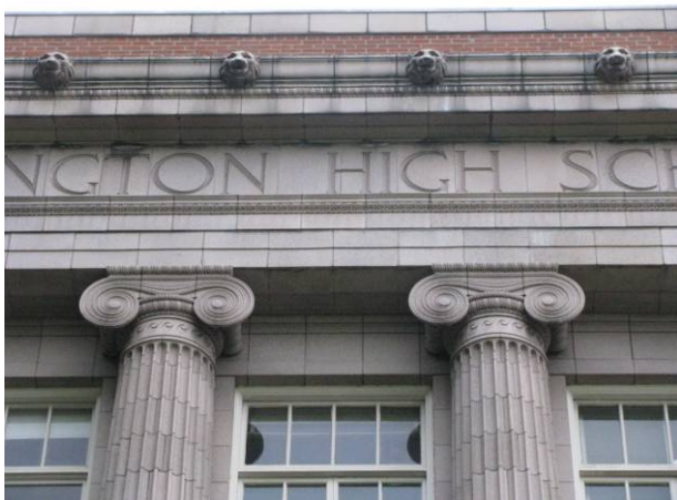
Main building (370A), detail of columns, looking east.
