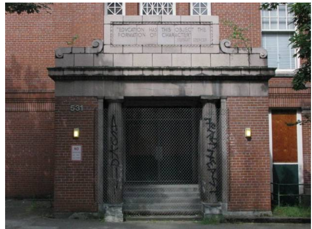
Main building (370A) rear (east) entry into building, looking west.
