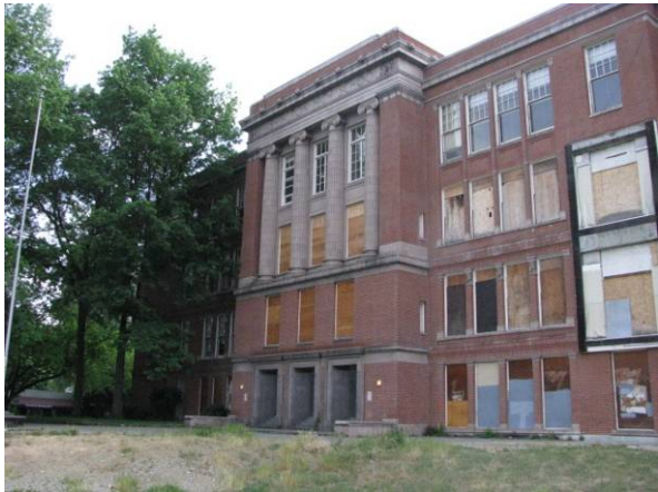
Main building (370A), looking northeast at principal elevation.
