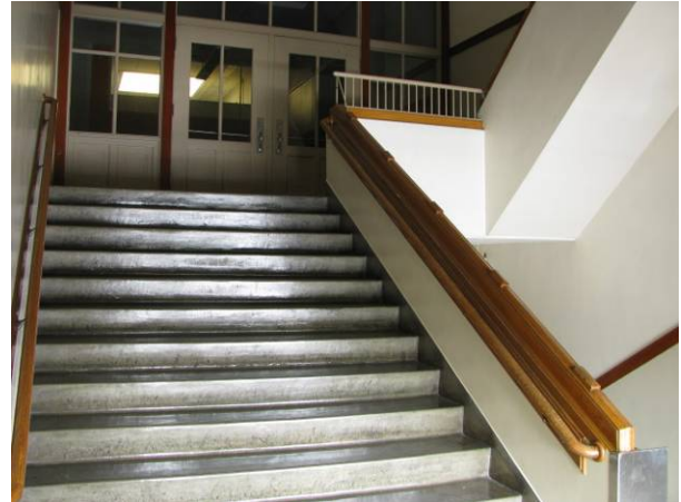
Main Building (370A), detail of staircase.
