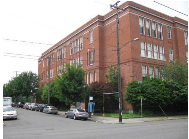
Main building (370A), looking southwest.
