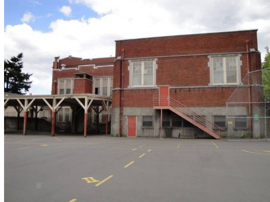
West elevation (and covered play shed)
