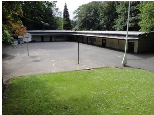
Classroom Annex east and south elevations
