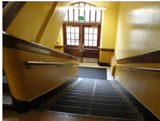
Stairwell facing south
