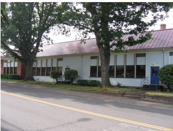
South elevation facing north
