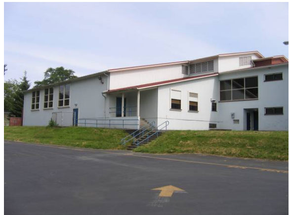
North elevation facing south
