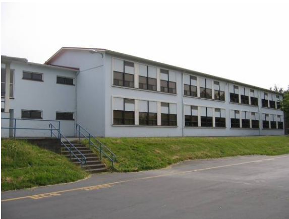
North elevation facing south
