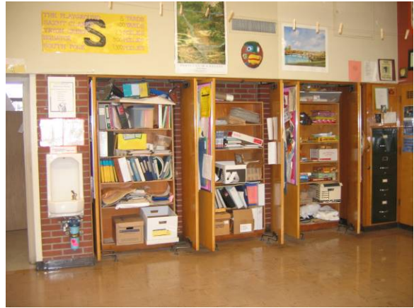
Classroom built-ins and exposed brick
