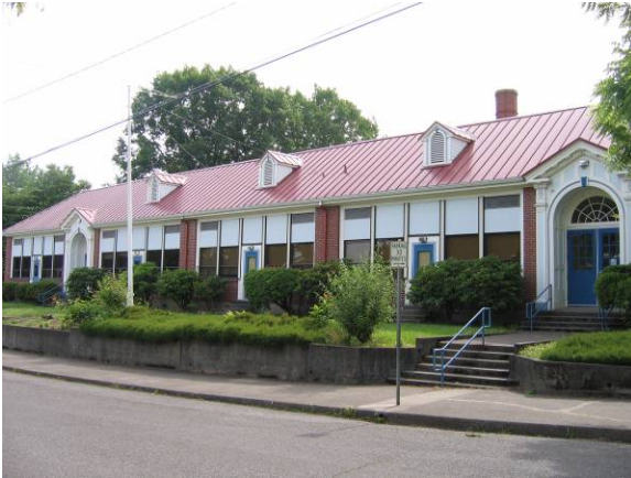
East elevation facing southwest
