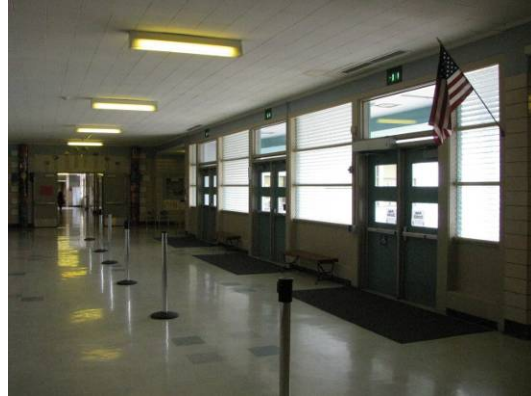
Main lobby (243A)
