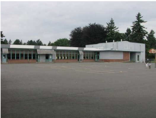
Main building, looking toward gymnasium (243A)
