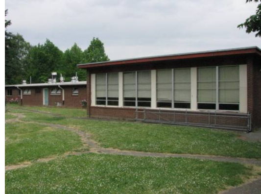
Creston Annex (243B) looking north.
