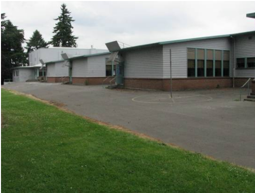
Main building, west classrooms (243A)
