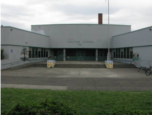
South elevation, main entrance (243A)
