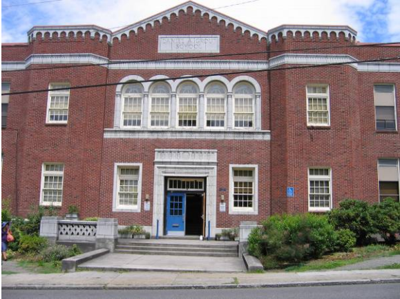
South elevation facing north
