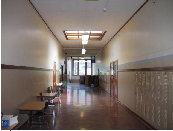
2 nd floor corridor and skylight
