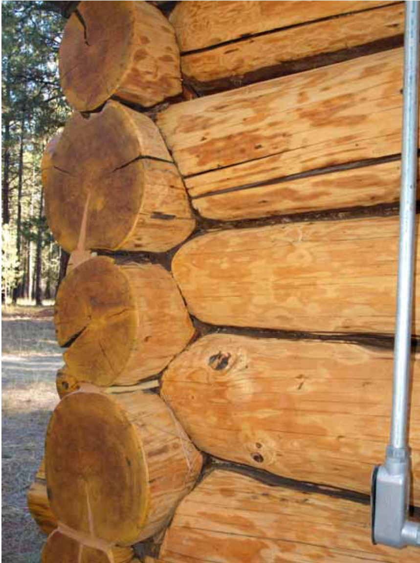
Photo 9 Detail, corner joints
