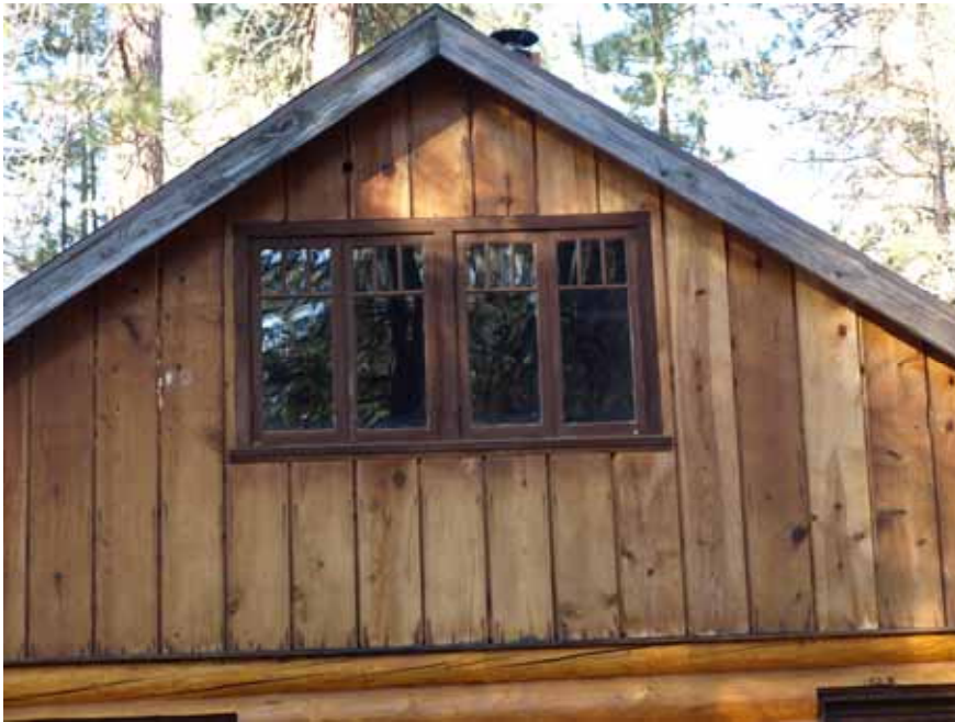
Photo 7 Casement windows, east elevation
