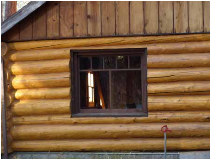
Photo 8 Fixed window, east elevation
