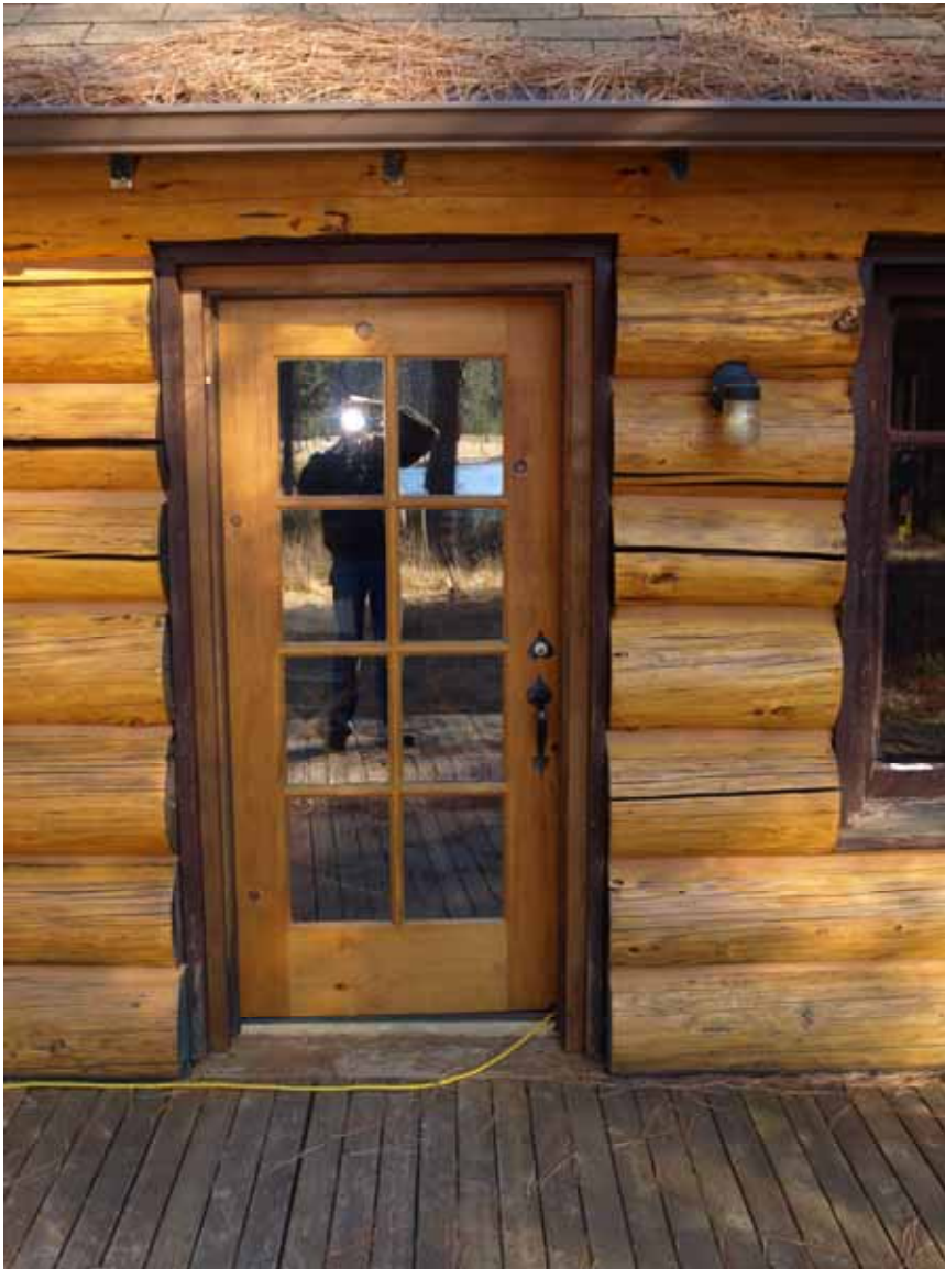
Photo 10 Detail, entry door
