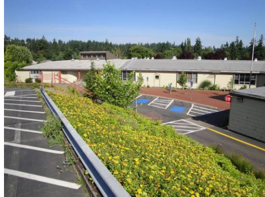
Southeast elevation; upper and lower parking areas
