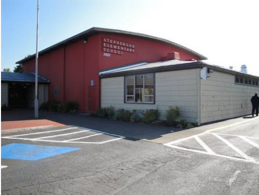
South (gymnasium) and west elevations
