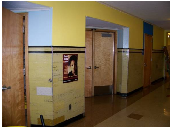
Main building (180A), restroom entrances, looking northwest.
