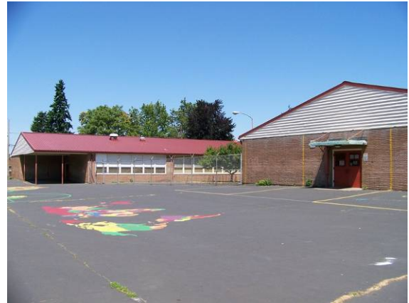
Main building (180A), south (rear) elevation of building wings, looking northwest.
