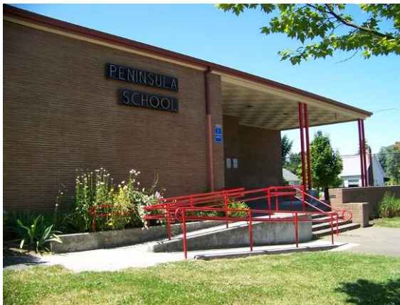
Main building (180A), north (front) elevation, looking southwest.
