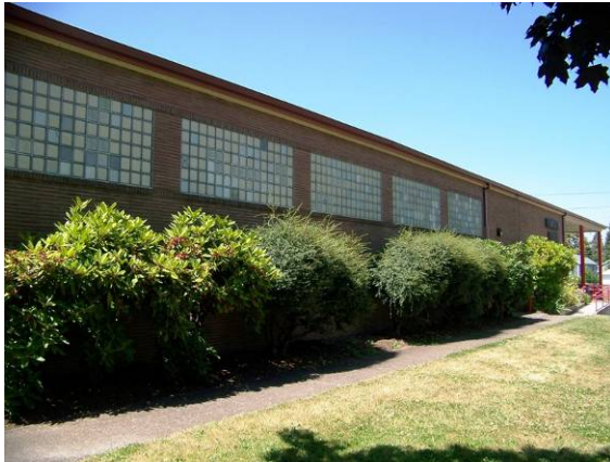
Main building (180A), north (front) elevation, looking west.
