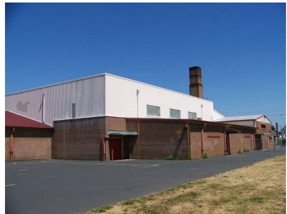
Main building (180A), east (side) elevation at the gymnasium, looking northwest.
