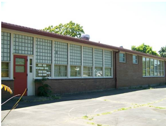
Main building (180A), west (side) elevation, looking southeast.
