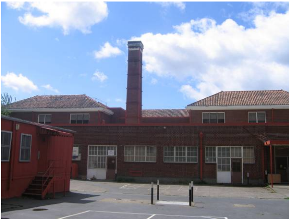
North elevation facing south
