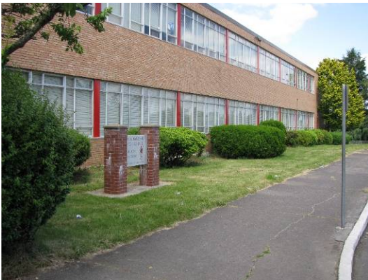
East elevation near main entrance (220A)
