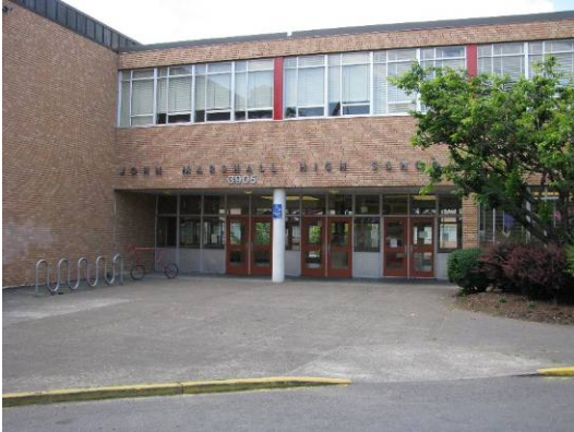
Main entrance, east elevation (220A).
