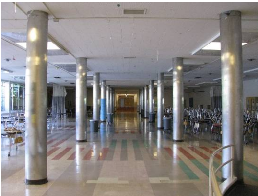
Cafeteria detail of structural columns.
