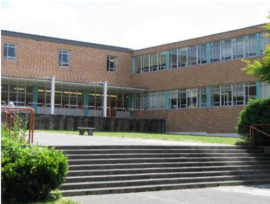
Interior courtyard, looking southeast (220A).
