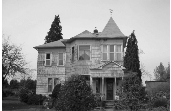
The Mill Keeper's House, 2005
