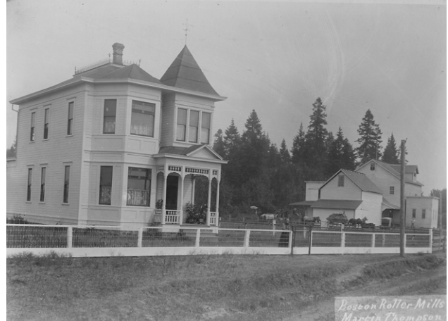
Mill Keeper's House, c 1904
