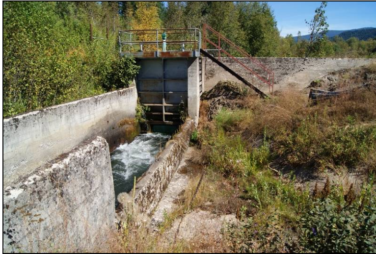
Figure 11. Red Blanket intake, canal, and lateral spillway, 2009.
