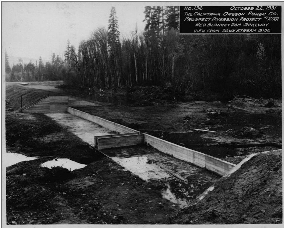
Figure 30. COPCO Prospect Diversion Project No. 2001, Photo No. 136, Red Blanket Dam Spillway, view from downstream side, October 22, 1931.
