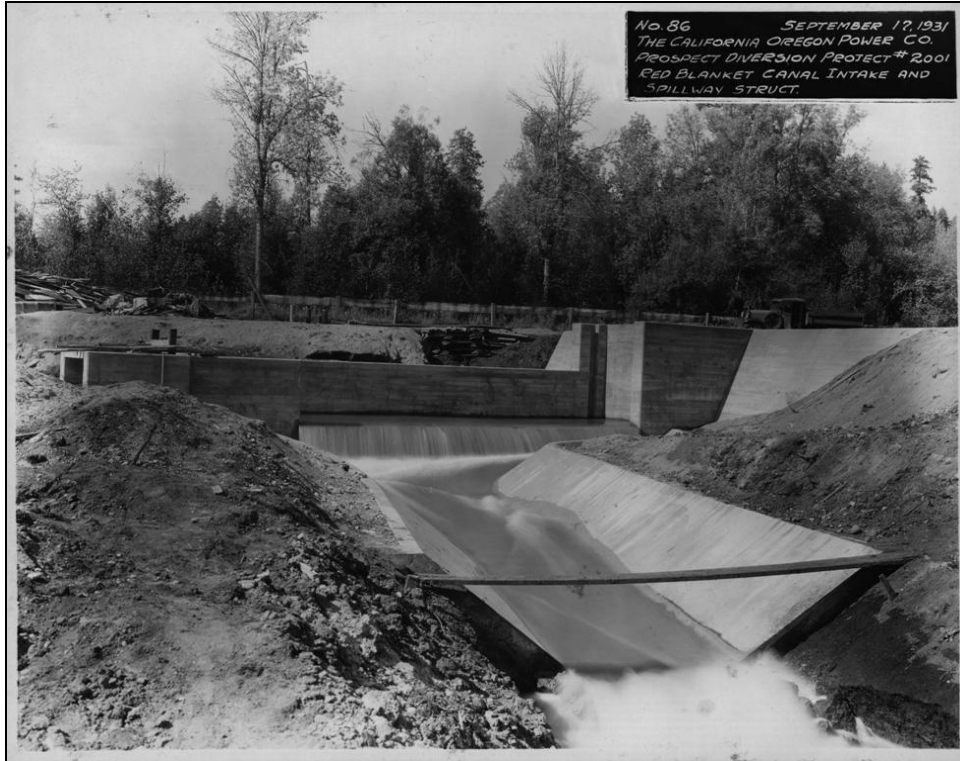
Figure 25. COPCO Prospect Diversion Project No. 2001, Photo No. 86, Red Blanket Canal Intake and Spillway Structure, September 17, 1931.
