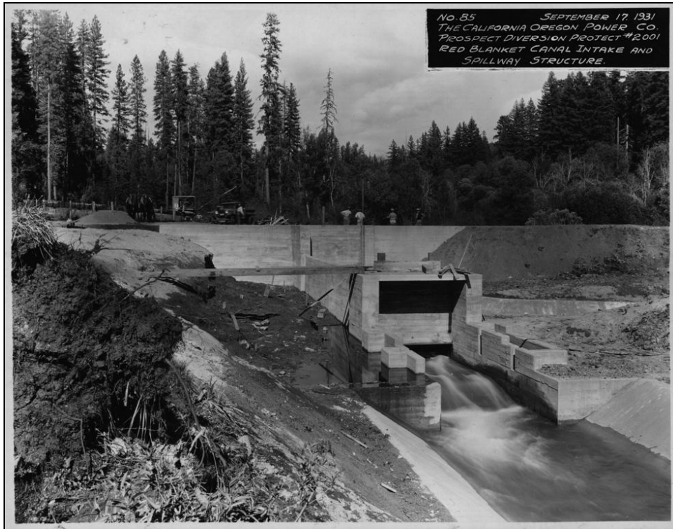
Figure 24. COPCO Prospect Diversion Project No. 2001, Photo No. 85, Red Blanket Canal Intake and Spillway Structure, September 17, 1931.
