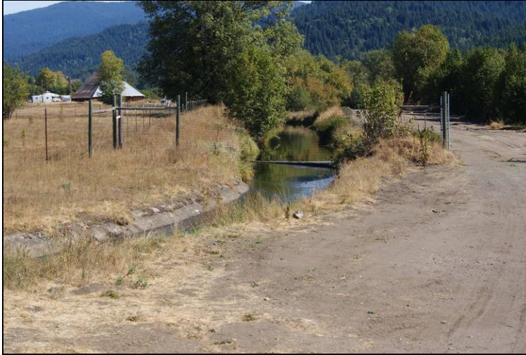
Figure 9. Red Blanket canal at intersection of unlined and lined segments just before Red Blanket canal merges with Middle Fork canal, 2009.
