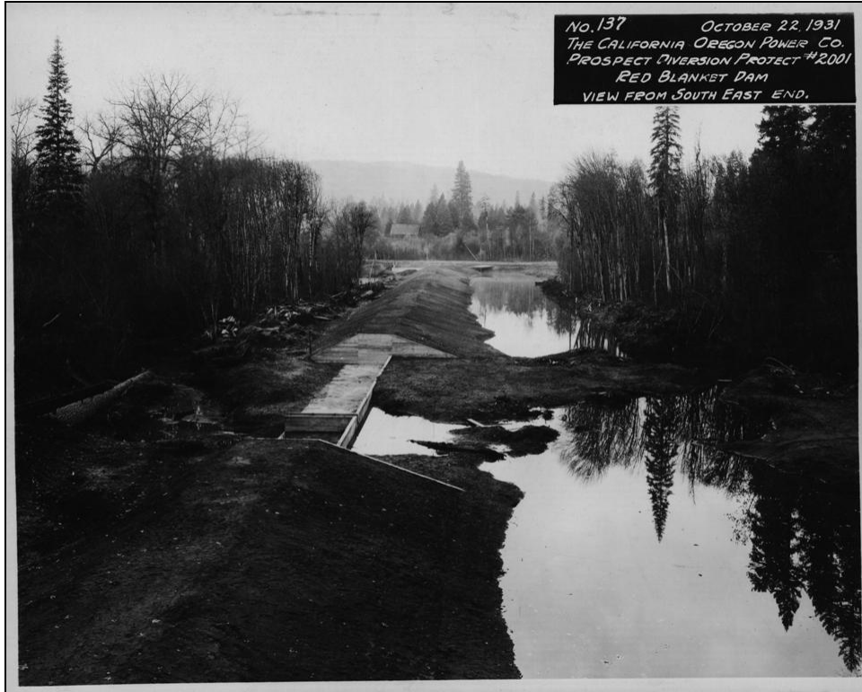
Figure 31. COPCO Prospect Diversion Project No. 2001, Photo No. 137, Red Blanket Dam, View from southeast end, October 22, 1931.
