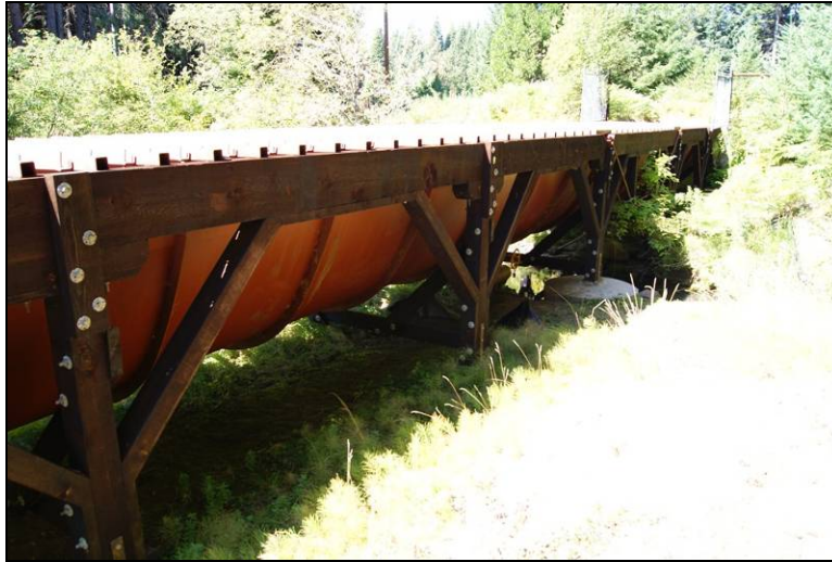
Figure 13. Steel flume on wooden trestle, downstream of Barr Creek gauge shelter, 2009.
