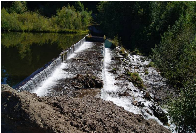
Figure 10. Red Blanket dam, 2009.
