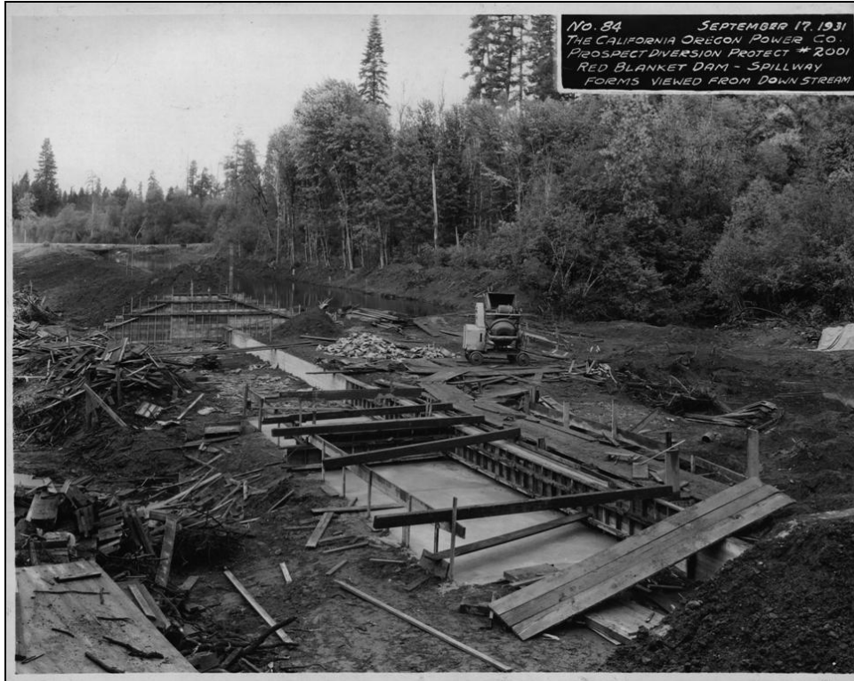
Figure 23. COPCO Prospect Diversion Project No. 2001, Photo No. 84, Red Blanket Dam – Spillway, forms viewed from downstream, September 17, 1931.
