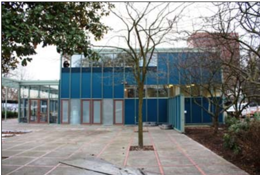
6 of 15: (OR_MultnomahCounty_VisitorsInformationCenter_0005.tif) North building elevation, looking south from courtyard.
