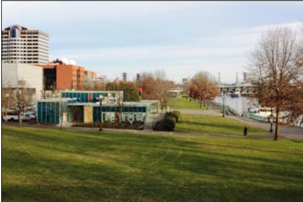
1 of 15: (OR_MultnomahCounty_VisitorsInformationCenter_0001.tif) Visitors Information Center viewed from Hawthorne Bridge, looking north.
