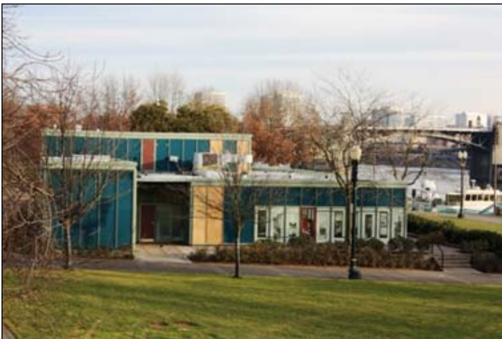
4 of 15: (OR_MultnomahCounty_VisitorsInformationCenter_0004.tif) South building elevation, looking north.
