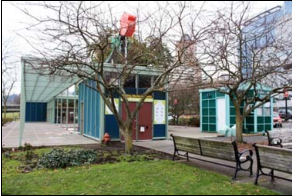
7 of 15: (OR_MultnomahCounty_VisitorsInformationCenter_0007.tif) North garden shed elevation, looking southwest.
