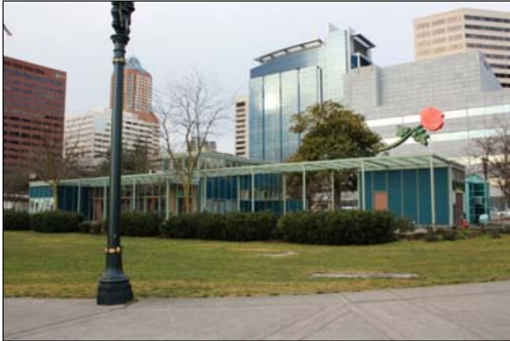
5 of 15: (OR_MultnomahCounty_VisitorsInformationCenter_0005.tif) East building elevation, looking southwest.
