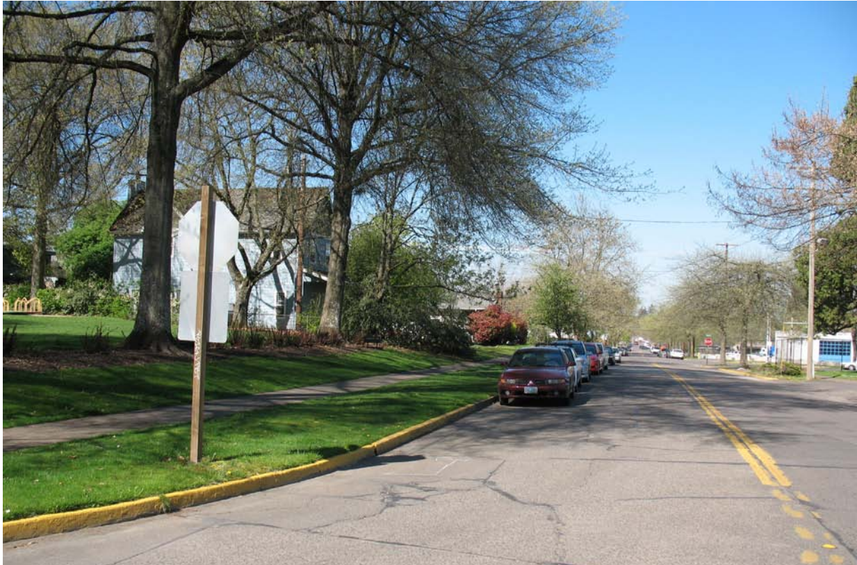
15th Avenue looking west
