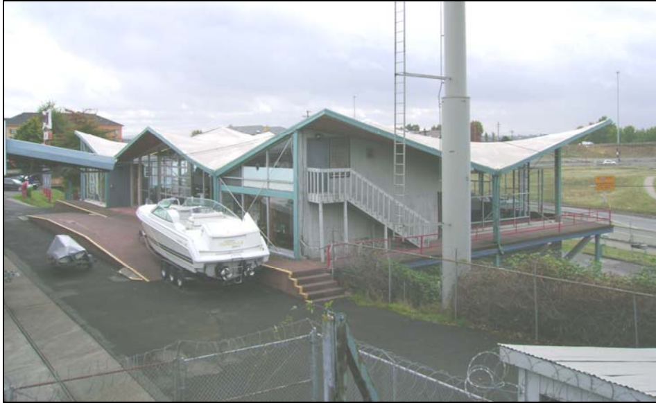
Figure 1: Looking south east at the north and west facades of the Totem Pole Marina building.
