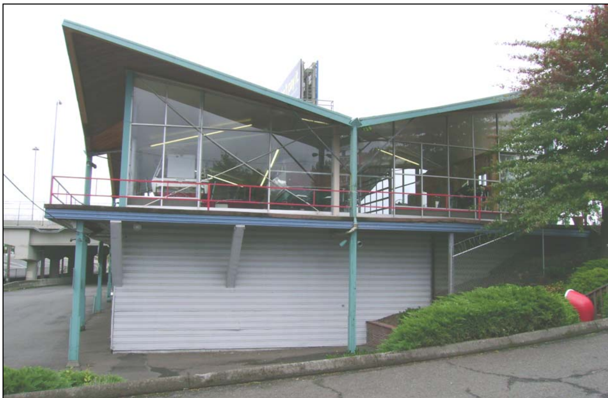
Figure 4. Looking west from the drive way on the east side of the building going toward the river.
