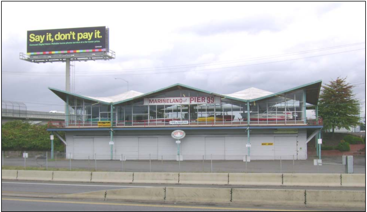
Figure 3. View: Looking north from Marine Drive, note I 5 overpass on the left side.
