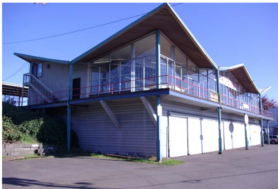
View of the south west façade of the Pier 99 Marine building, 1441 N. Marine Drive. Photo by Dan Wise November 2007
