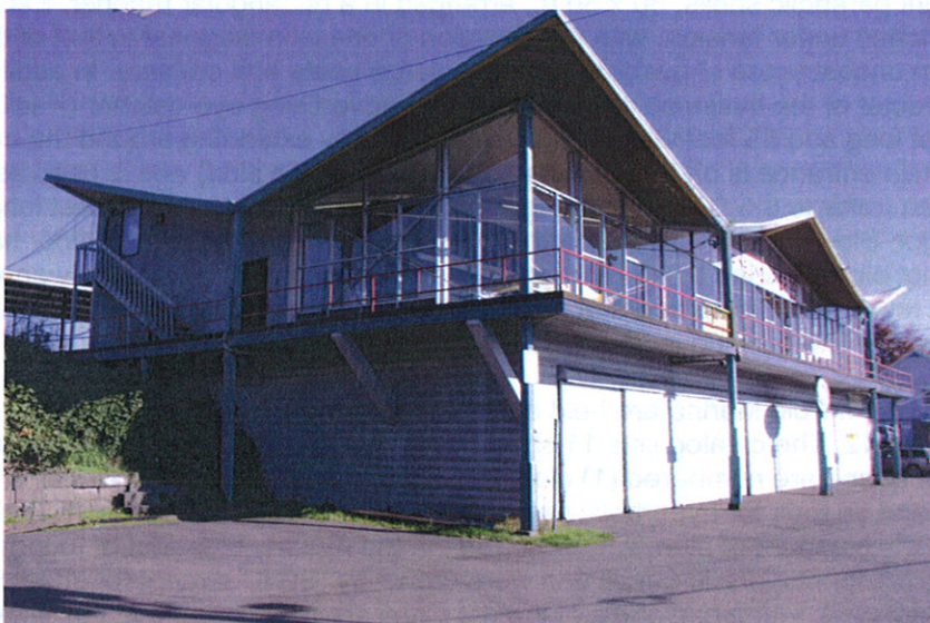
View of the south west façade of the Totem Pole Marina (Pier 99) building, 1441 N. Marine Drive. Photo by Dan Wise November 2007
