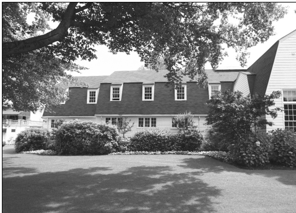
OR_ClackamasCounty_WaverleyCountryClubClubhouse_0006 Exterior View, looking east at west façade of 1930 addition
