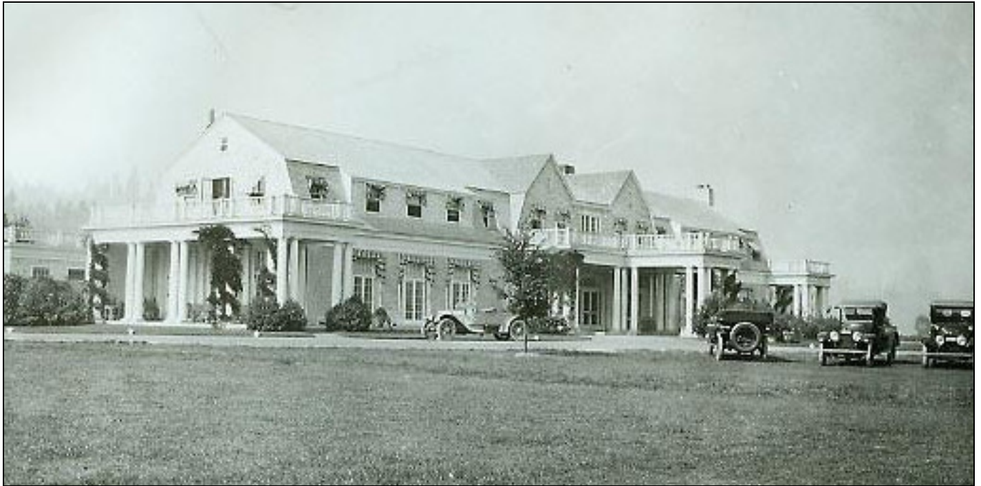
Figure 7: Photographs of Waverley Clubhouse, June 1913 (Top, looking NW; bottom, looking SE)
