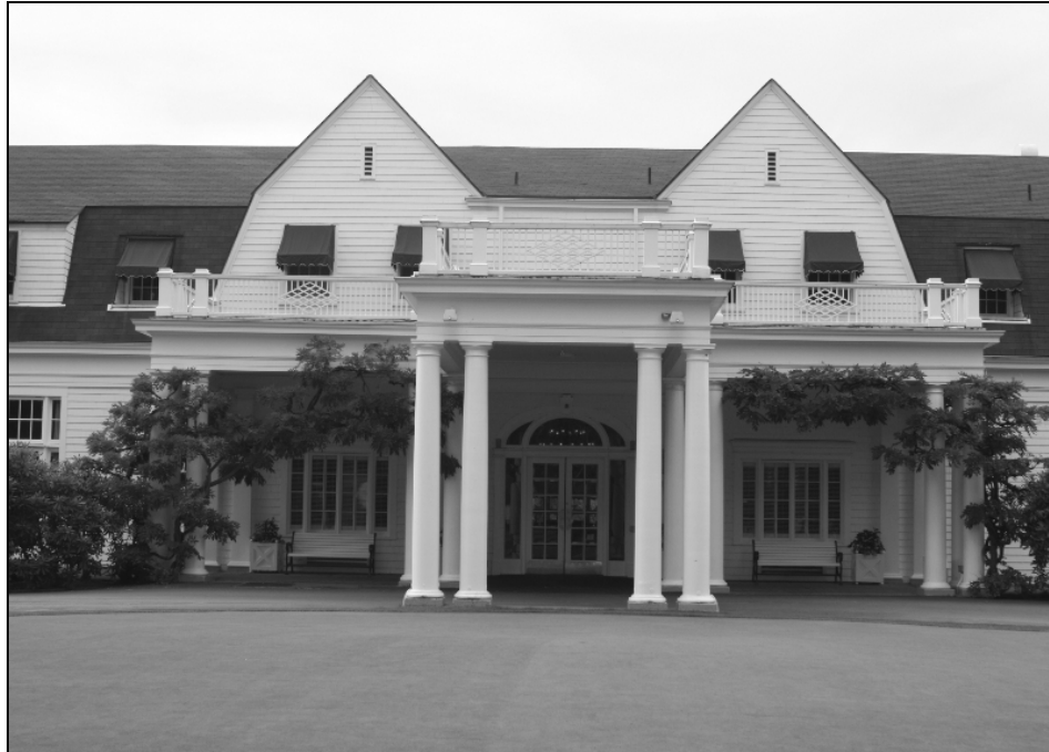
OR_ClackamasCounty_WaverleyCountryClubClubhouse_0003 Exterior View, looking west at east façade, main entry
