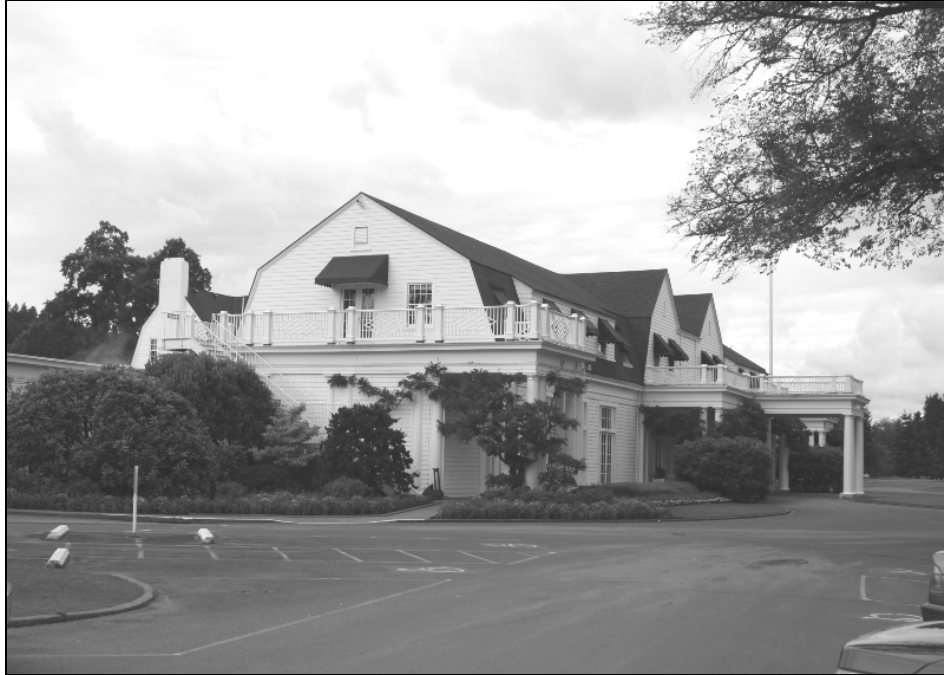
OR_ClackamasCounty_WaverleyCountryClubClubhouse_0009 Exterior View, looking northwest at south and east façade
