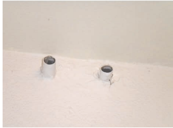
^ NORTH HALLWAY PIPE CUT OFF.
