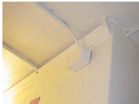
SOUTH HALLWAY MOLDING DETAIL. >
