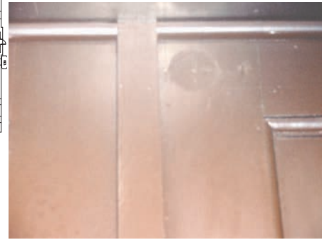
^ BATON AND BUMPER SCAR DETAIL.
