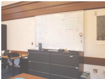
^ FURNITURE BLOCKED WEST DOORWAY.
