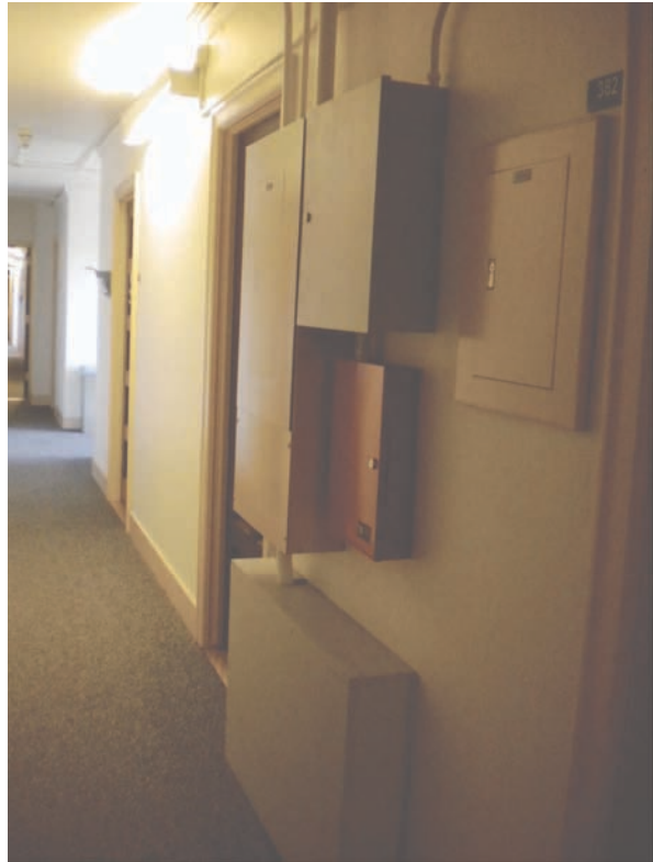
^ SOUTH HALLWAY THIRD FLOOR.
