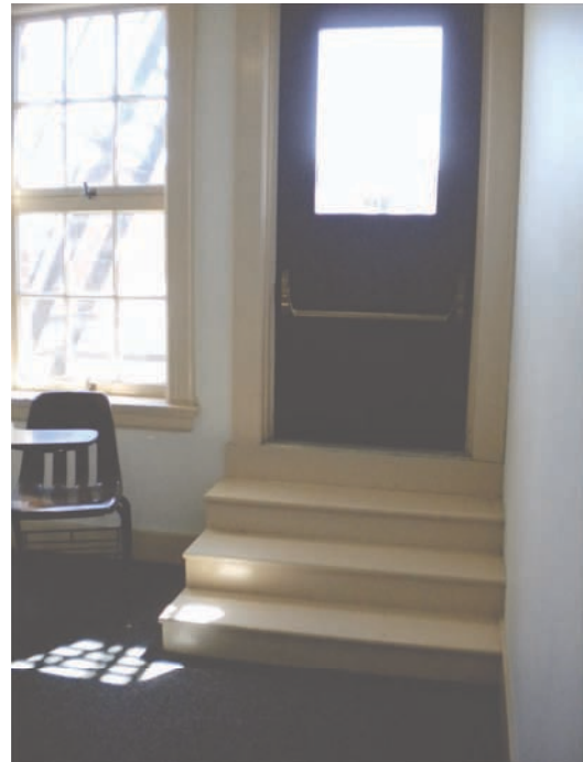
^ NORTH HALLWAY 3RD FLOOR FIRE ESCAPE.
