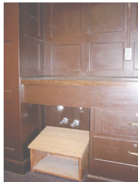
^ FORMER SINK STATION.
