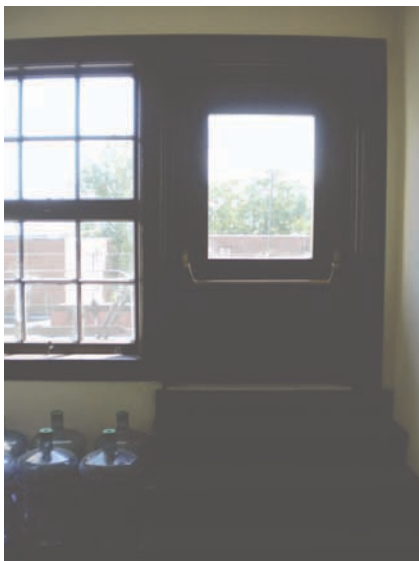
^ NORTH HALLWAY 4TH FLOOR FIRE ESCAPE.
