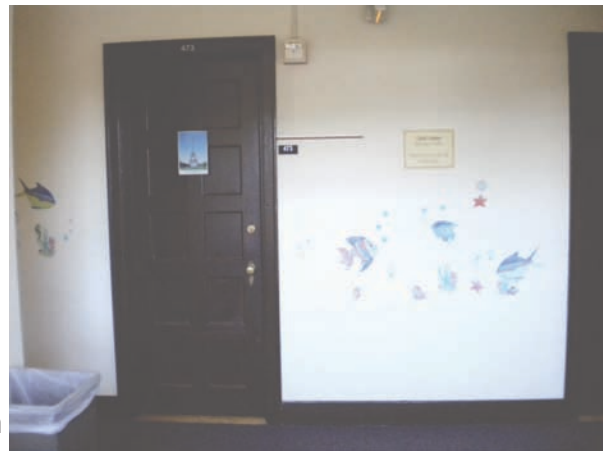
^ SOUTH HALLWAY 4TH FLOOR DETAIL.
