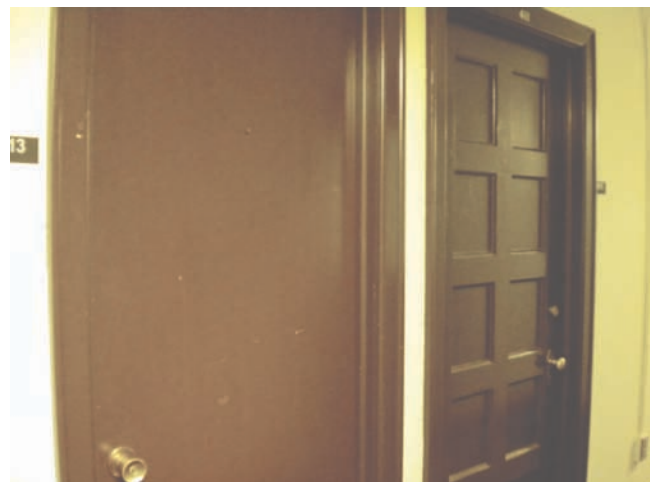
^ NORTH HALLWAY 4TH FLOOR NEW VS. OLD DOOR.
