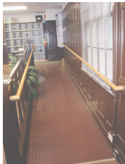
^ NEW RAMP AND WALL PANELS.
