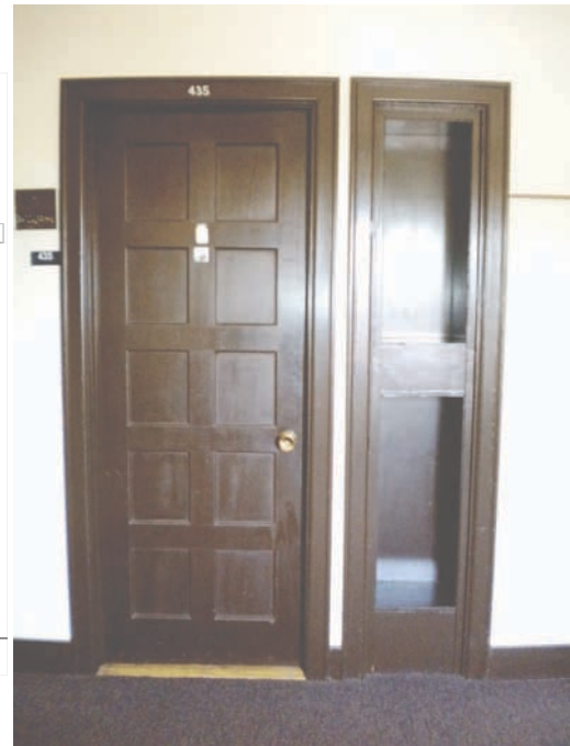
^ NORTH HALLWAY 4TH FLOOR ORIGINAL DOOR AND TELEPHONE CASE.
