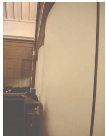
^ SOUTH WALL - ACOUSTICAL PANELS.
