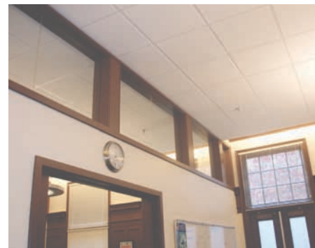
^ NEW PARTITION WALL.
