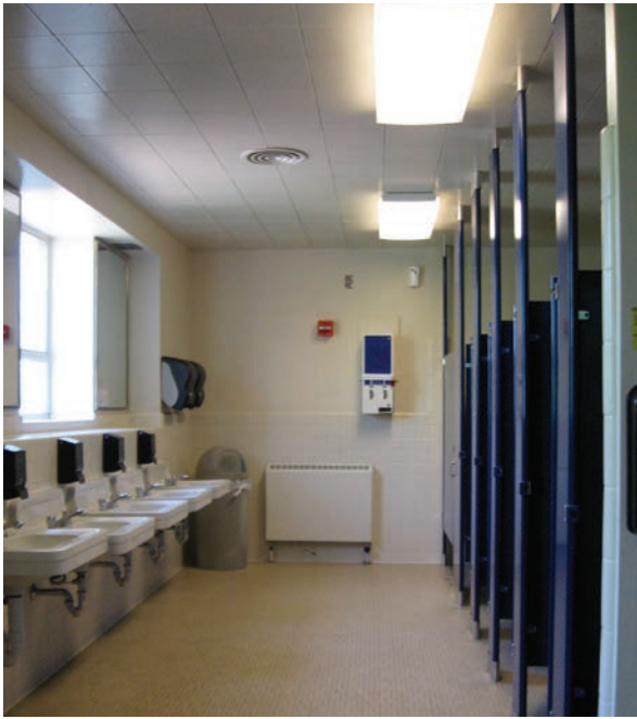
Women's Restroom (looking south).
