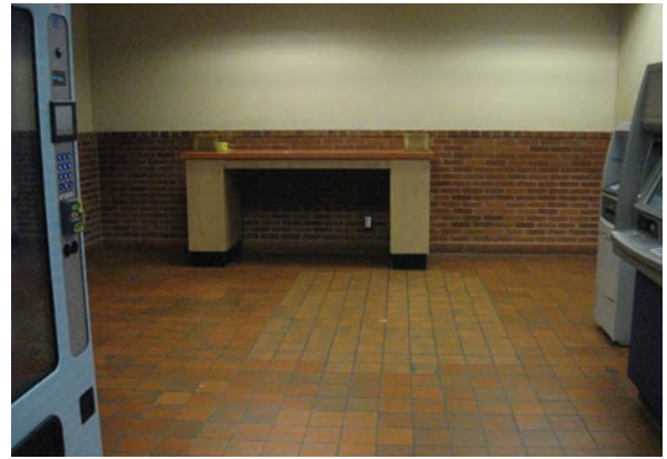
West wall - original brickwork.
