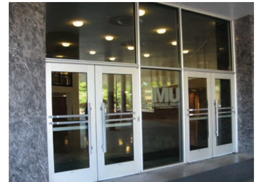
Main Entrance doors & windows replaced in 2009, maintaining hardware.
