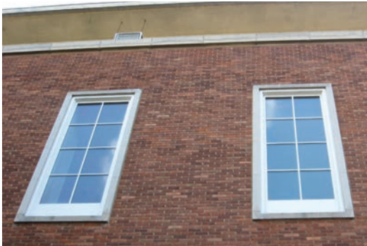
Second-floor windows had glass replaced in 2009; original wood frame & mullions.
