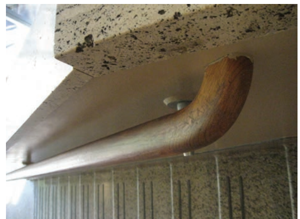
Hallway (looking north).
