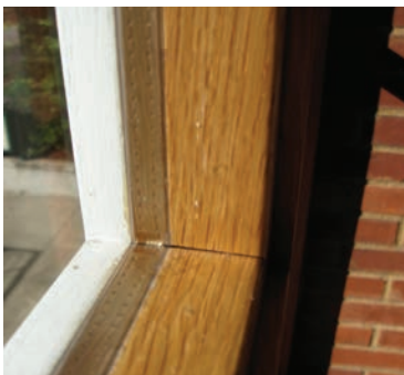
Detail of routing to fit second pane of glass in original hardwood windows.
