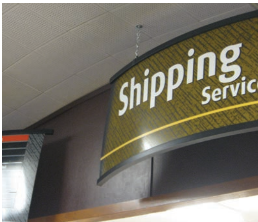
Curved ceiling above wood fascia
