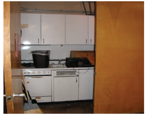
Original kitchenette on south wall.
