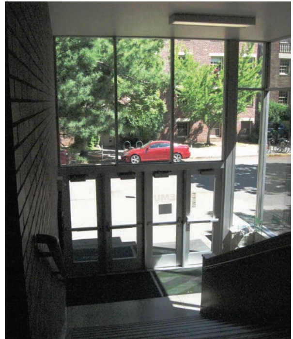
South Entrance Stair, original windows & aluminum storefront.
