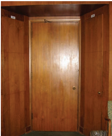
Original entry to the Boardroom on east wall. Original walnut veneer panels & door hardware.
