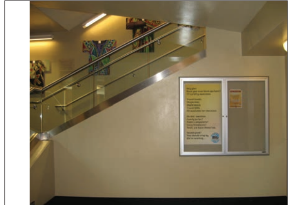
New handrails installed in 2000 Mills International Center remodel (looking north).
