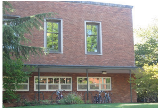
Second-floor windows all replaced in 2007.
