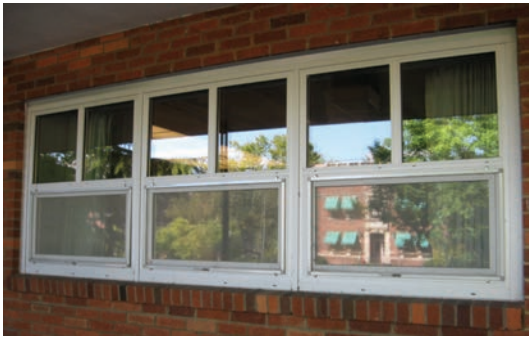
All north-facing windows in the Walnut Room were replaced in 2009. A wider opening was cut for windows, date unknown.
