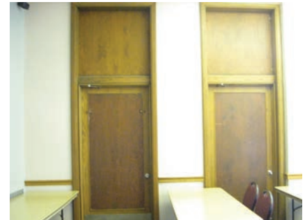
Interior view of original doors from Maple Room to second floor balcony, closed off due to office expansion during the 1985 addition.
