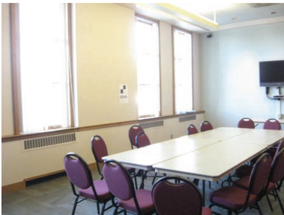
Single pane glass replaced with double pane in 2009.
