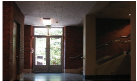
Glass panes in doors replaced in 2009 (looking west).
