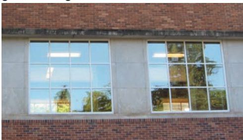
First-floor windows, glass replaced in 2009.
