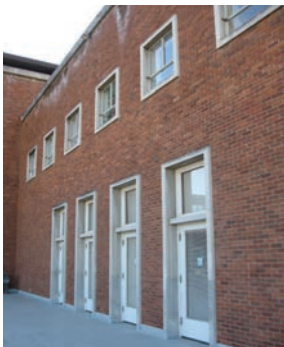
(2.) Three original balcony doors, with far right door retaining original hardware.
