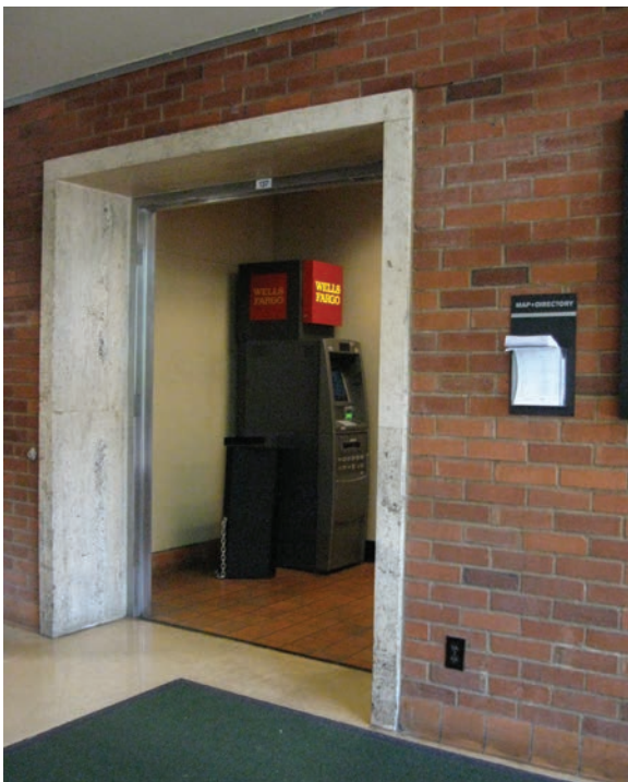
Looking south towards ATM Center.
