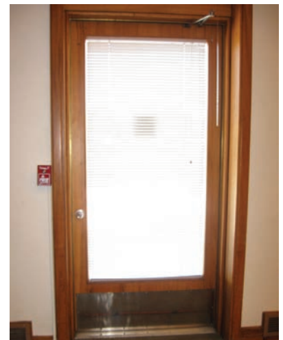
Remaining original hardware and door.
