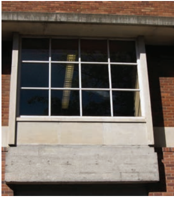
Original east windows of Taylor Lounge with original stone trim.
