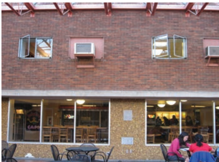
Original 1950 exterior wall converted to courtyard space (facing west).
