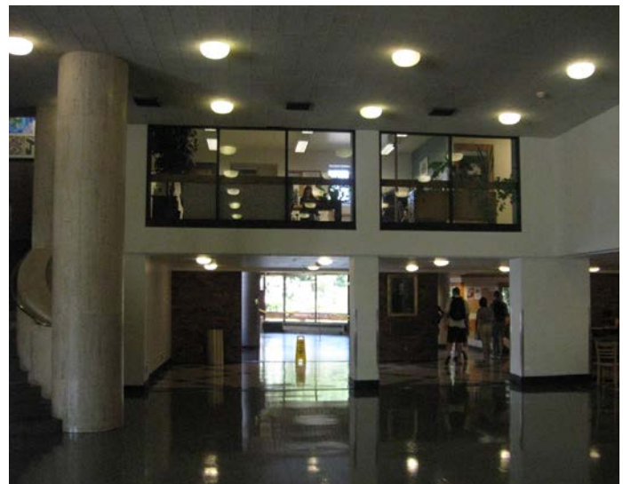
Looking east to 1970s addition - Mezzanine storefront windows added.
