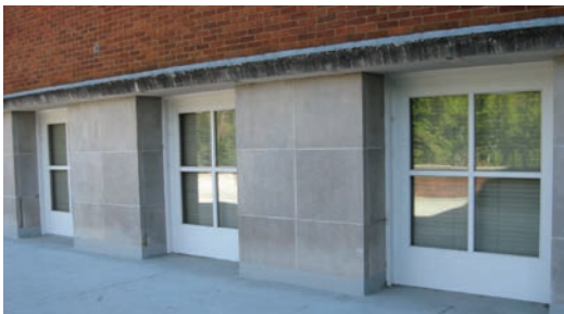
(3.) Three sets of double doors replaced by double-over-double windows in 1985.
