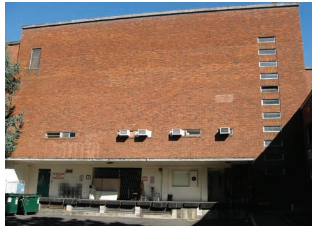
South loading zone with original windows & doors.
