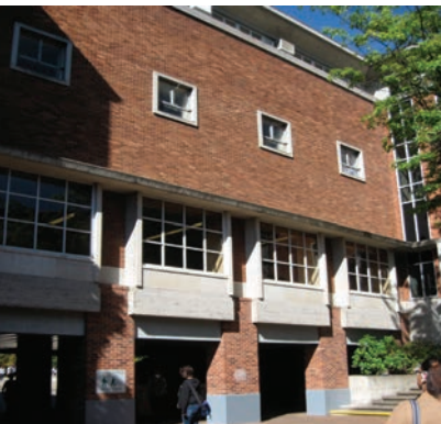
View from basement-level breezeway excavated in 1973.
