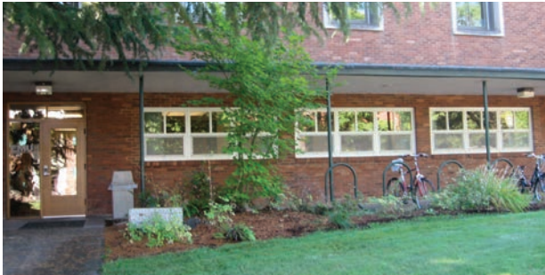
Original opening for Post Office double-swing door, replaced in 2009 with a single swing door.
