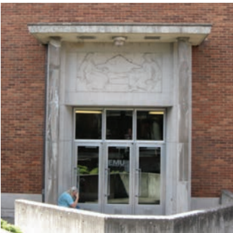
Original opening & engraving of East Entrance w/steel door and window replacements in 2009.
