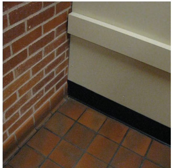
Original brick and quarry tile floor.
