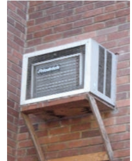
Infilled window far south edge of west wall, w/vent, date unknown.
