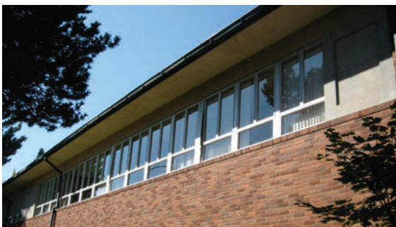
East-facing office windows replaced in 2009, with original stone panels (top right).
