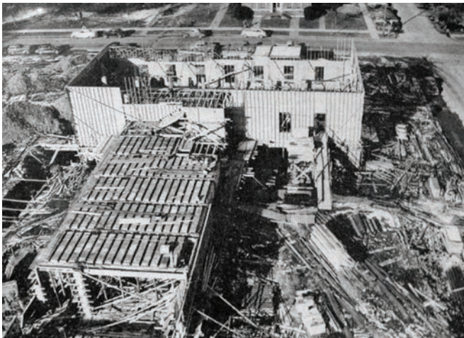
Aerial of the EMU under construction, c. 1949.
