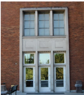
(1.) Replacement doors & hardware in 2009. Original cast concrete detailing & upper level windows.
