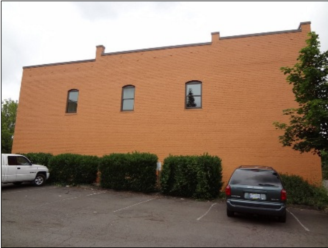
Photo 5 of 10: South facade, camera facing north.
