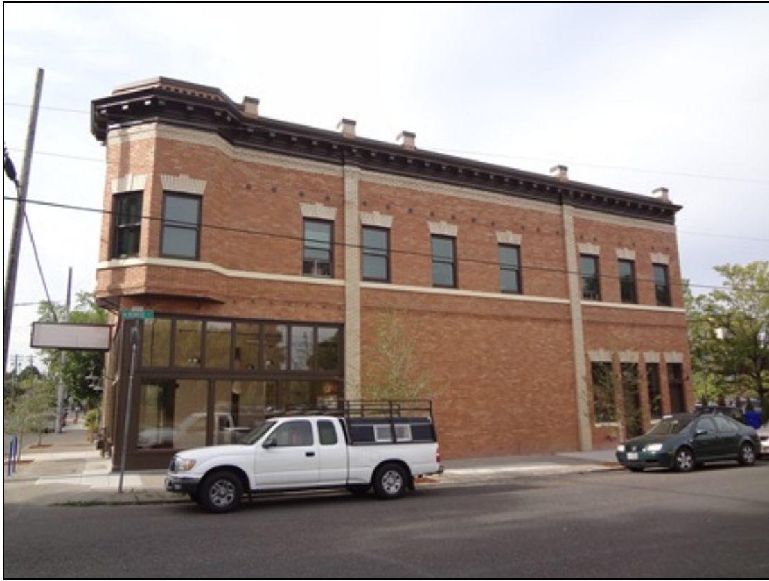
Photo 3 of 10: North facade, camera facing southwest.
