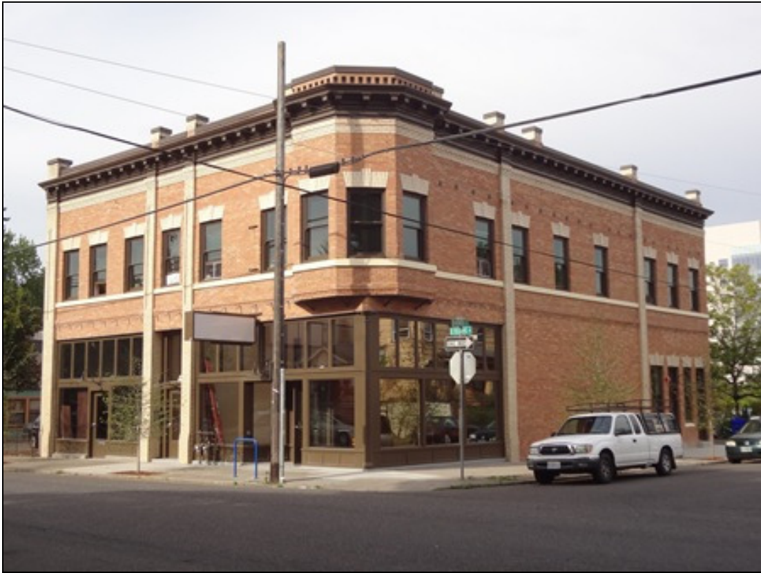
Photo 1 of 10: East and north facades, camera facing southwest.
