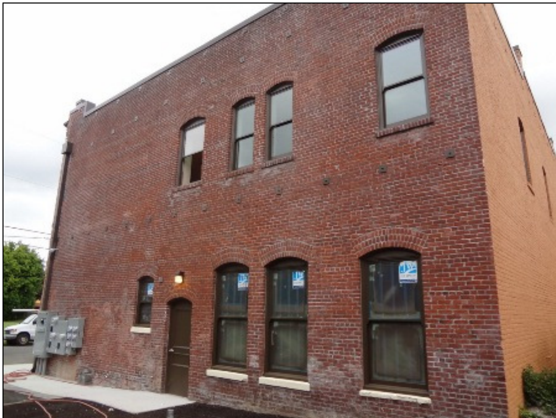
Photo 4 of 10: West facade, camera facing east.
