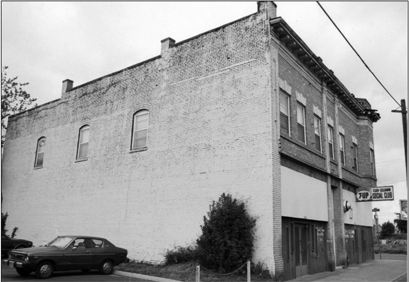
Figure 10: The Rinehart Building, approximately 1981 prior to the removal of its original cornice
