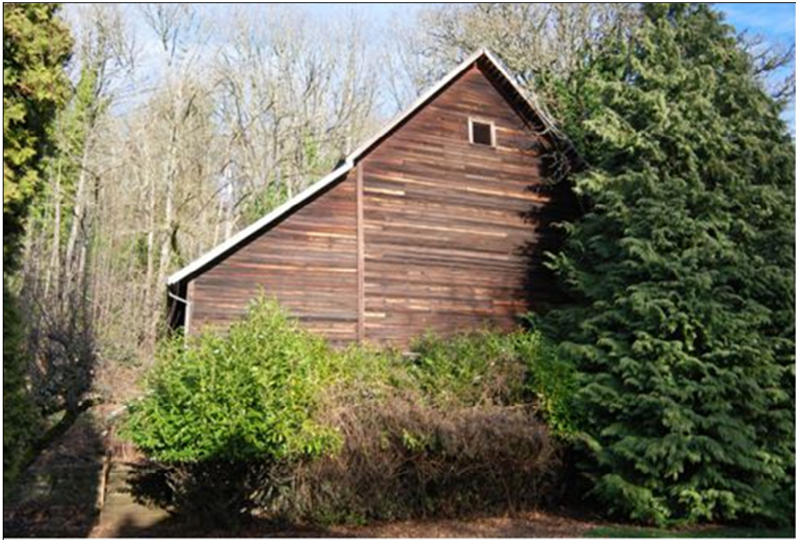
Photo 5 of 8: Looking east at the west façade.
