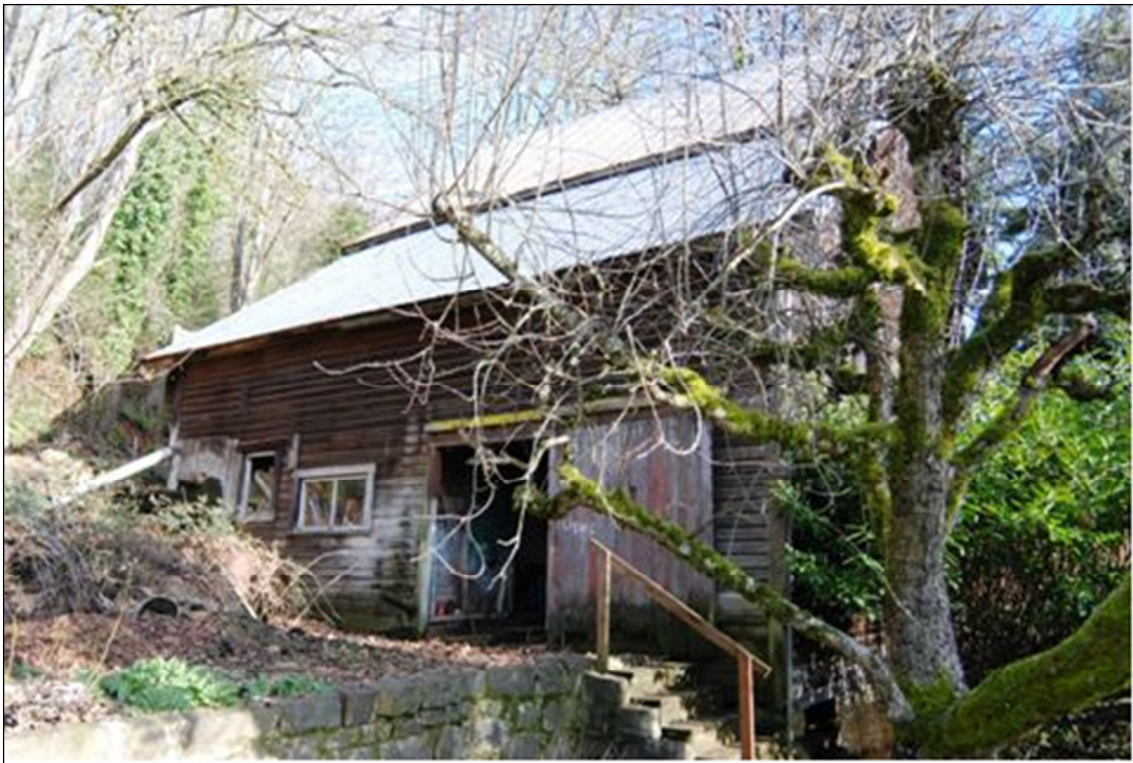
Photo 4 of 8: Looking southeast at the north façade.
