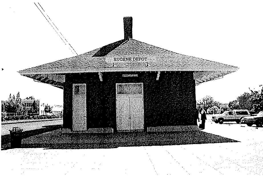
6. Looking east, west façade of depot.
