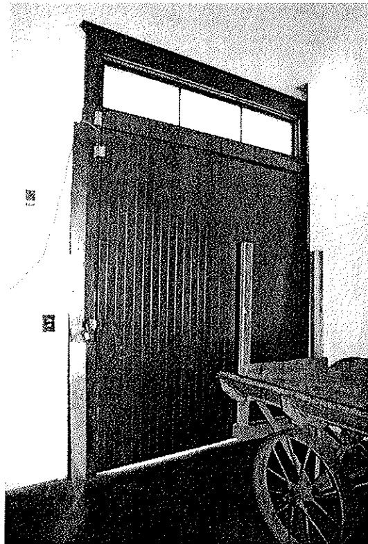
18. Looking southwest, interior of depot freight room, rolling freight door and door pocket.
