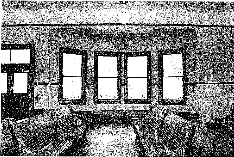
15. Looking north, interior of depot round bay window.
