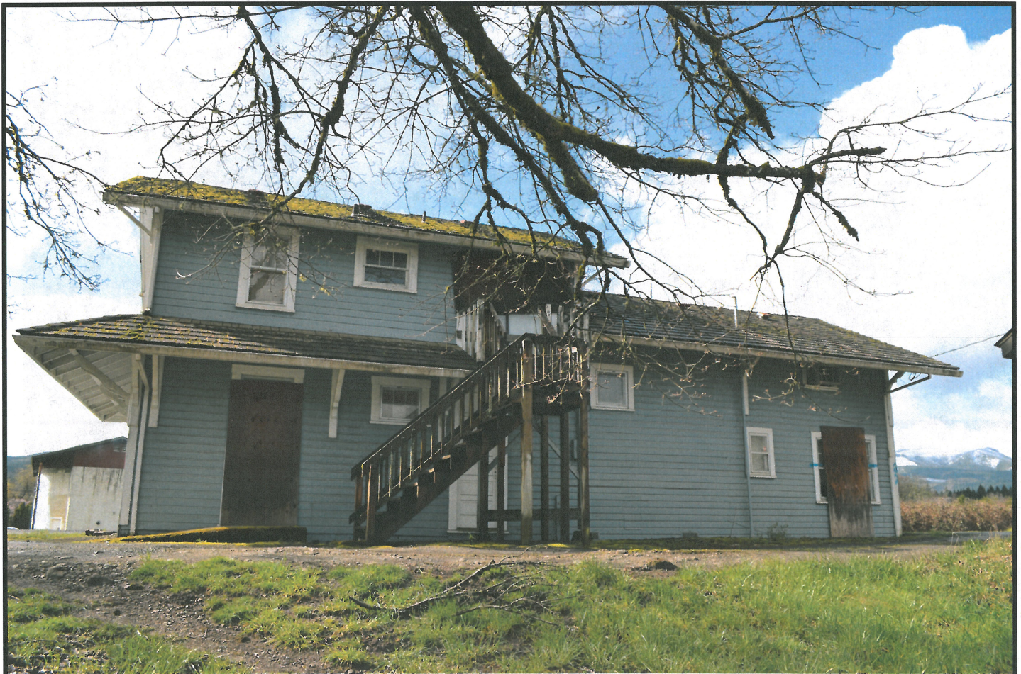
Photograph 6. Grand Ronde Rail Depot North Facing Façade showing emergency exit staircase.
