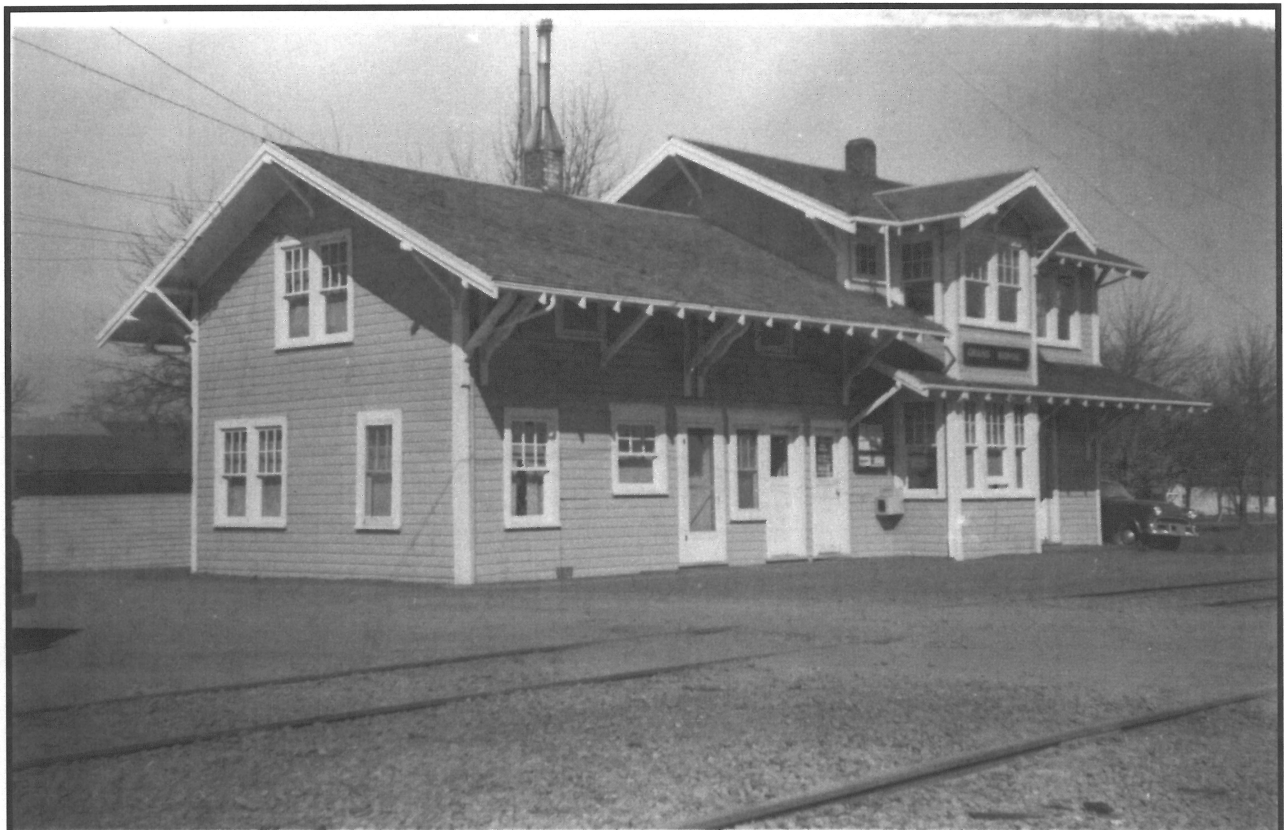
Photograph 2. "Grand Ronde Rail Depot
