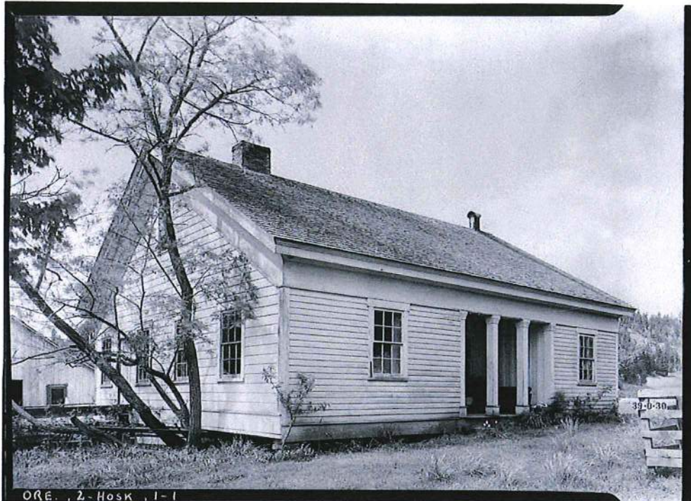
Figure 12. James and Mary Watson House, 1852, Kings Valley, Benton County. Image courtesy Historic American Building Survey.
