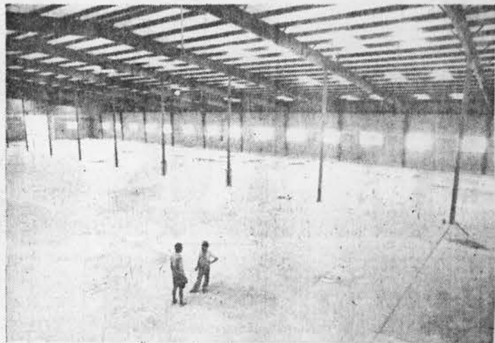
Interior view of one of the buildings at the Al Arda marketing complex.
