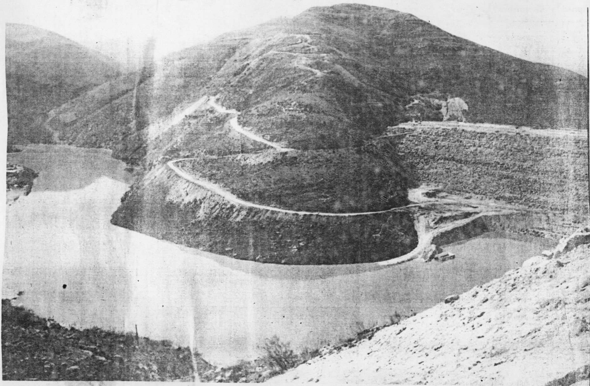
Water for irrigation in the Jordan Valley is stored in the reservoir of the King Talal Dam.
