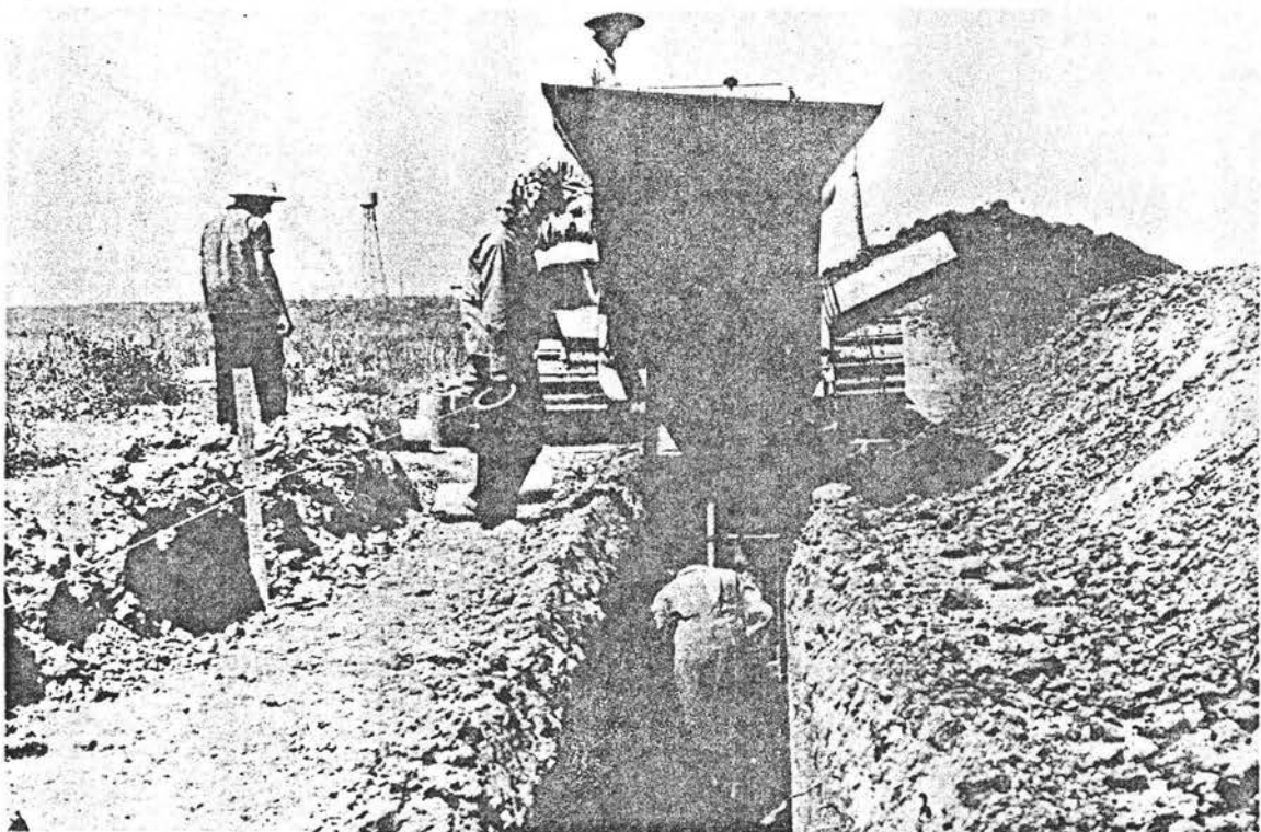
Plate 2 Cleveland trencher and crew laying pipes at Seyhan Project
