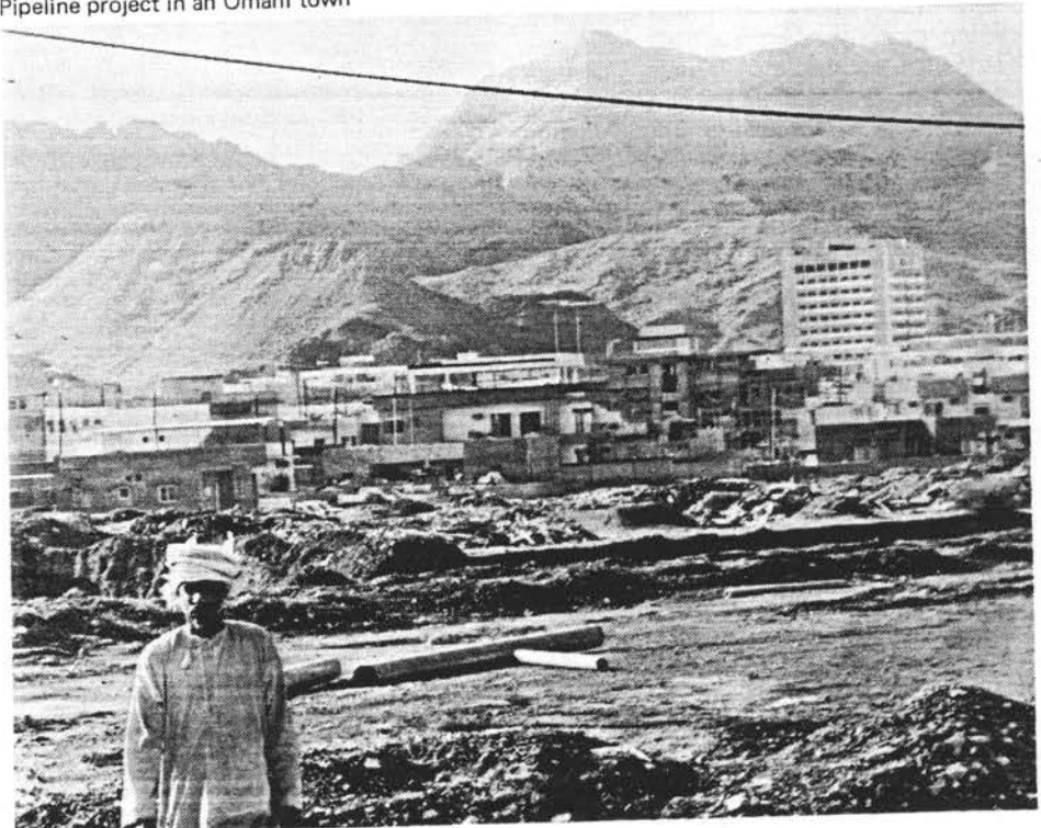
Pipeline project in an Omani town
