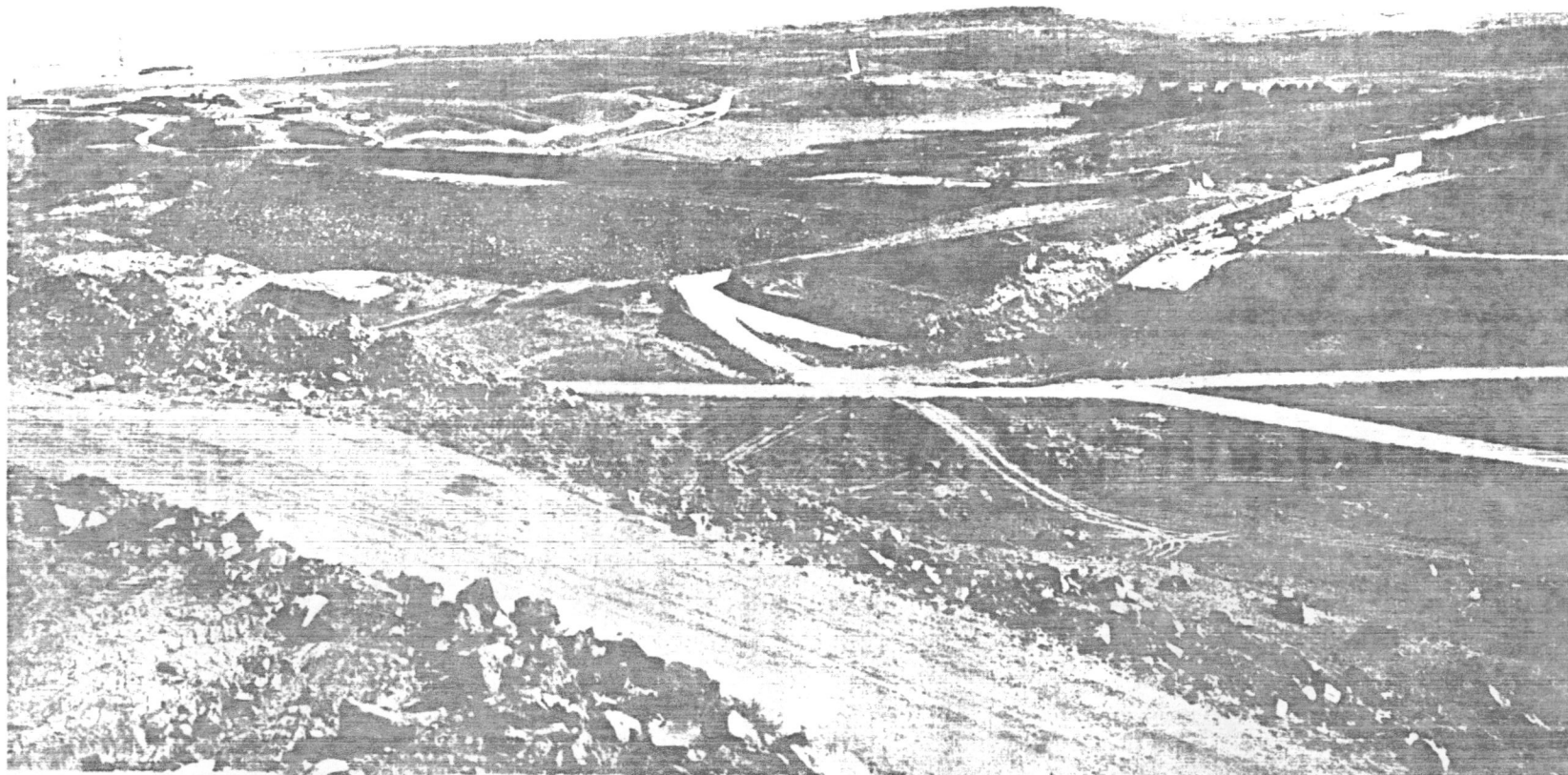
Fig. 5.001 Construction of the embankment and the spillway, Sarmisaklı Dam.
