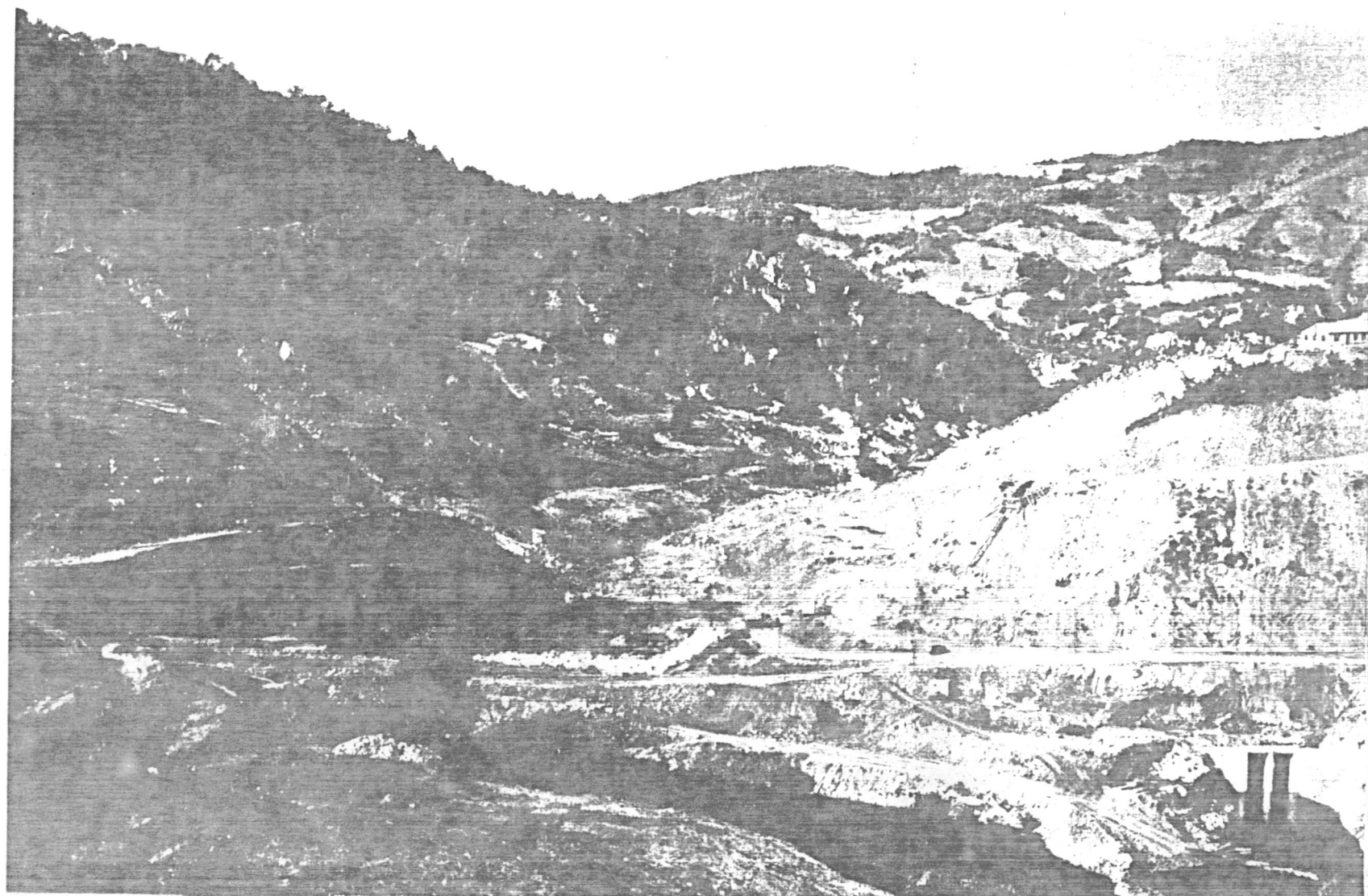
Fig. 5.017 Upstream view of the site, Hasanlar Dam.
