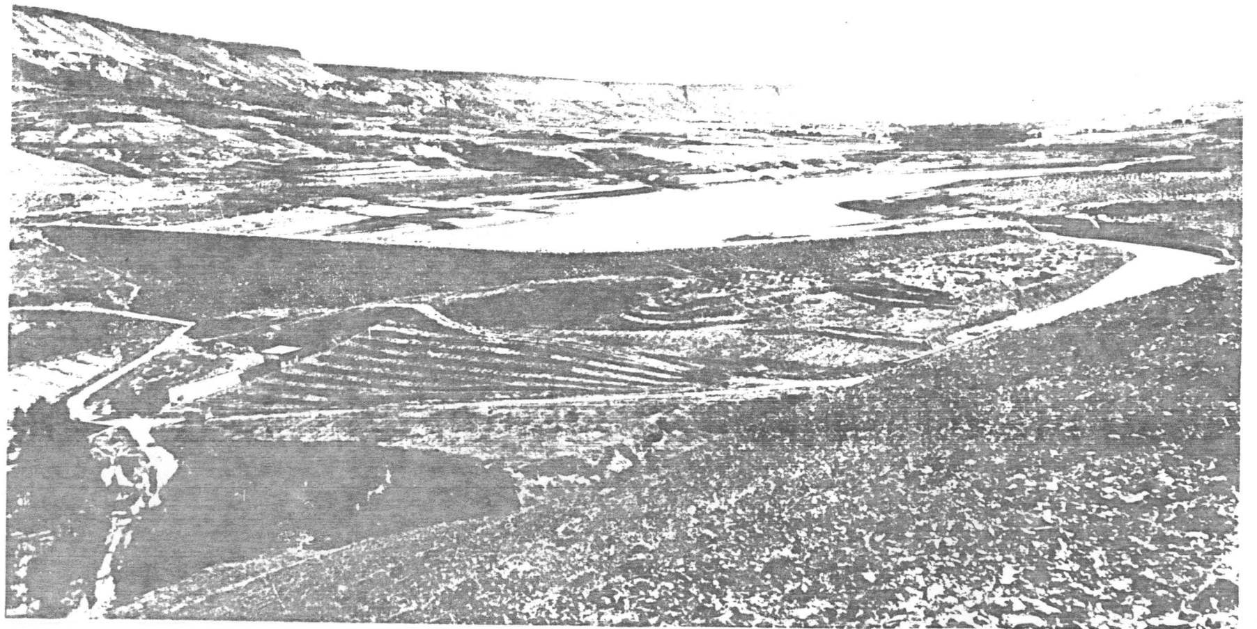
Fig. 3.05 General view of Damsa Dam.
