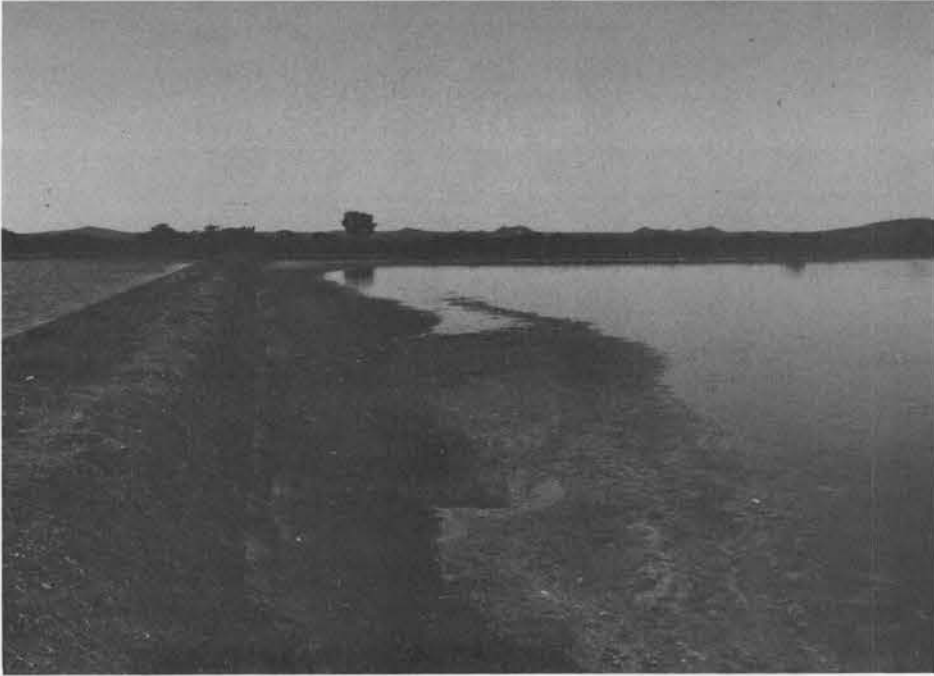
Figure 6. Embankment protection using precast-concrete slabs and pond drying for sludge removal.
