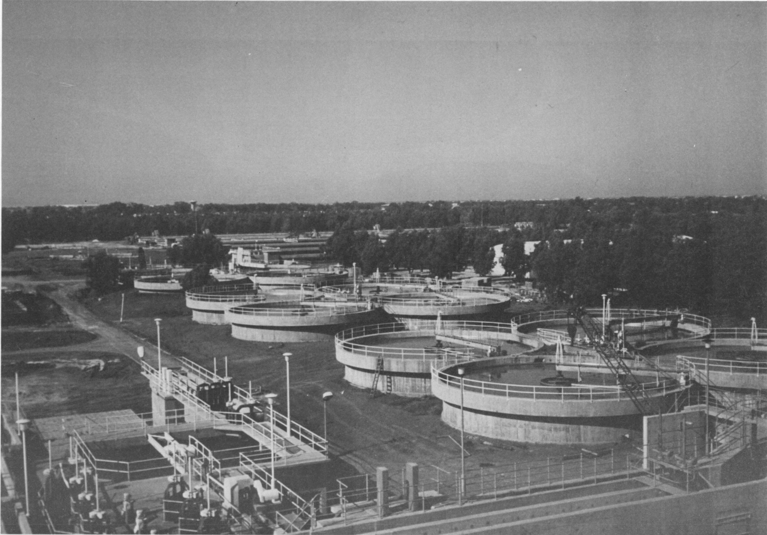
Figure 2 Primary sedimentation tanks at Guarchia Sewage Treatment Works Benghazi, Libya.
