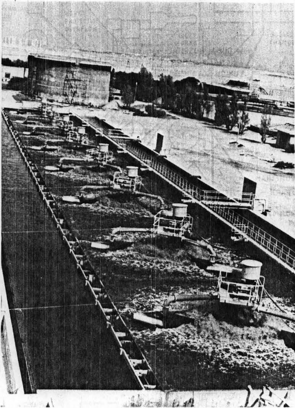
FIGURE 10 The aeration lagoon before modification
