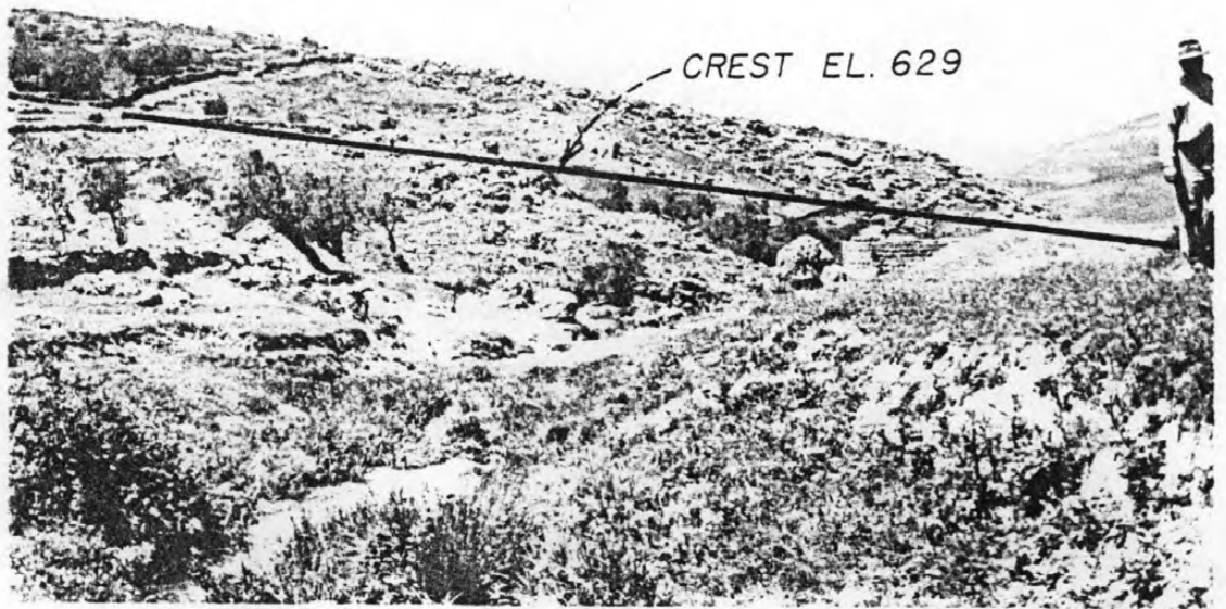
Kelia Forebay Dam Site - Looking Downstream
