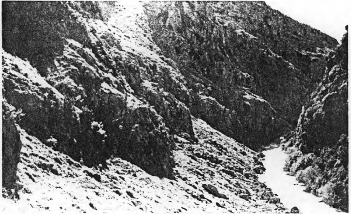
Narrow Litani River Canyon above Kelia Power Plant Site Looking Downstream
