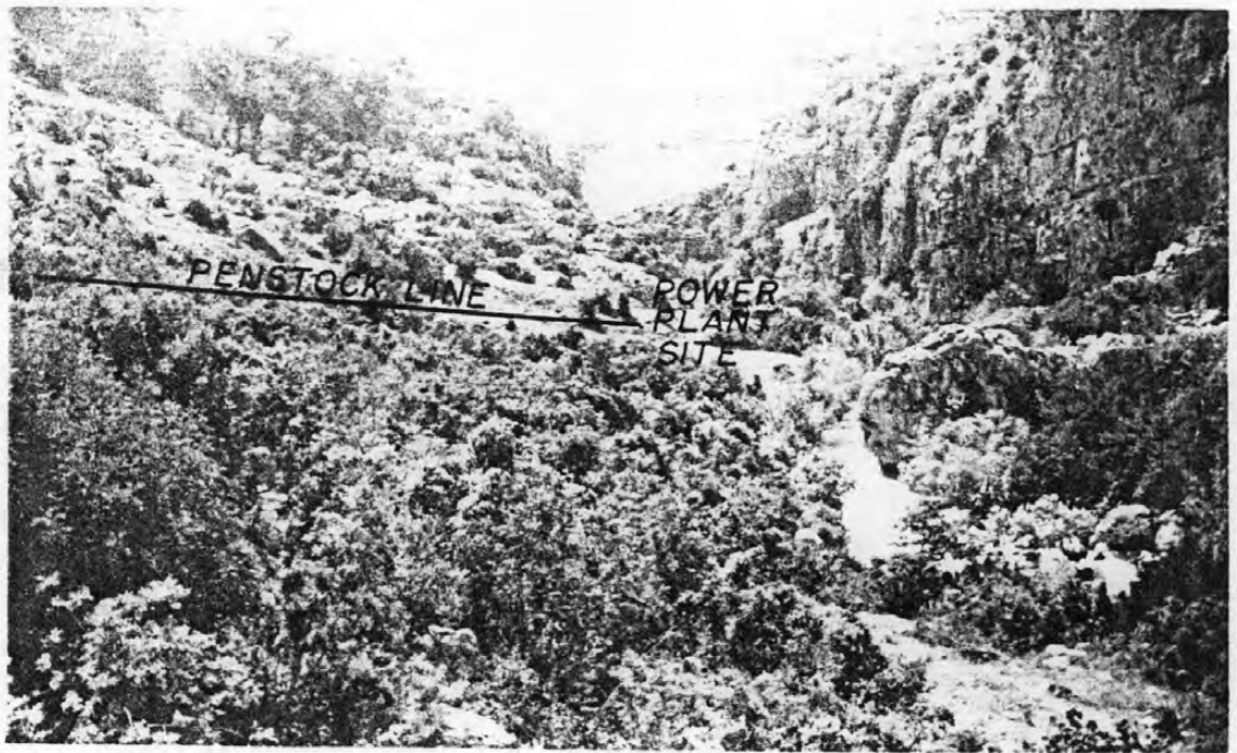
Kelia Power Plant Site - Looking Downstream
