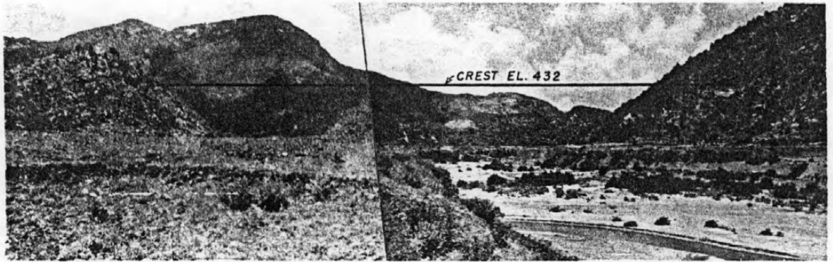
Bisri Dam - Axis B - Looking Downstream
