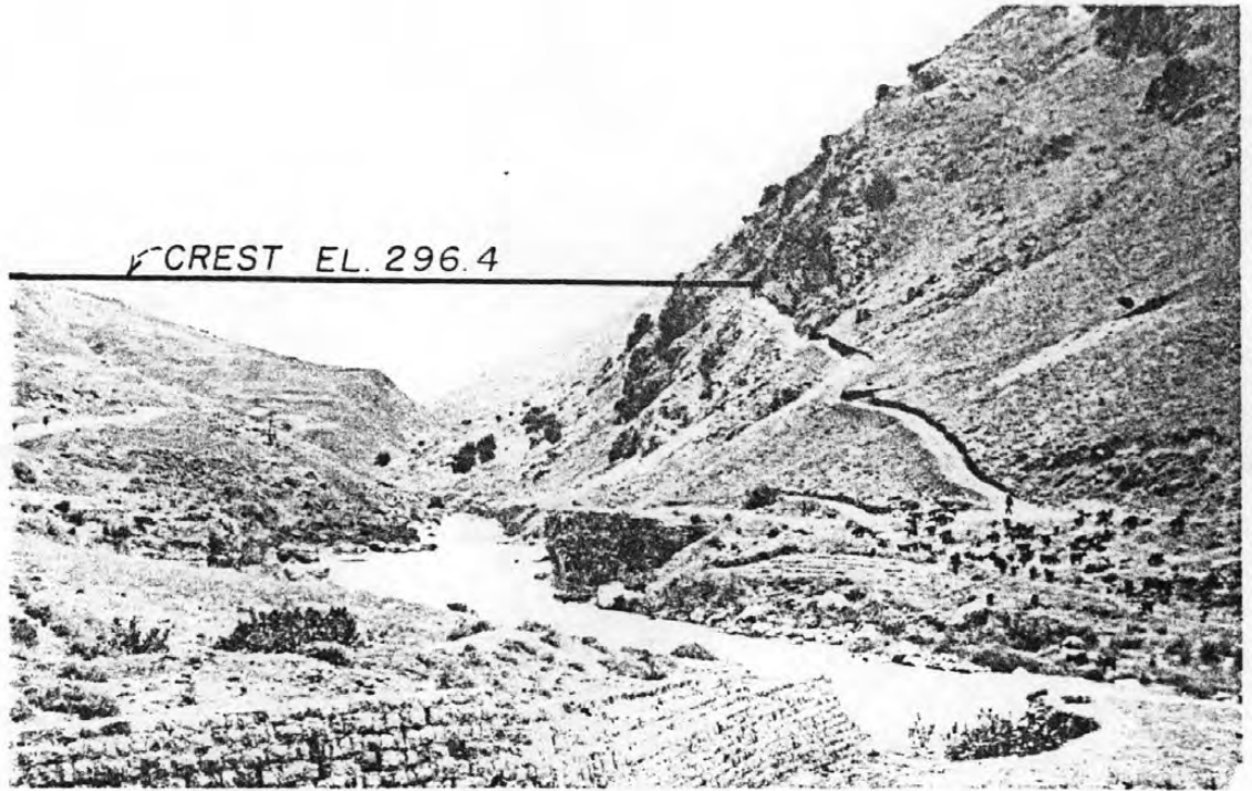
Khardale Dam site - Looking Downstream
