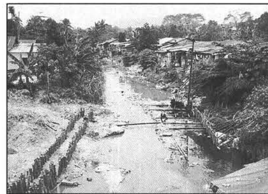
Above, an ineffective effort at controlling riverbank erosion through the placement of logs.
