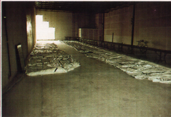
Prototype bag 100m long, 5000t displacement under construction.
