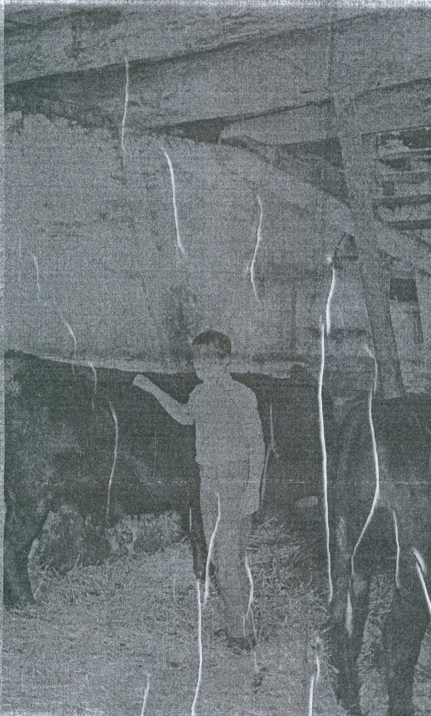
FOUNDATION WALL, HAND BUILT, 22 inches thick, supports the sturdy Elligsen barn where son Rudie tends his County Fair entry.
