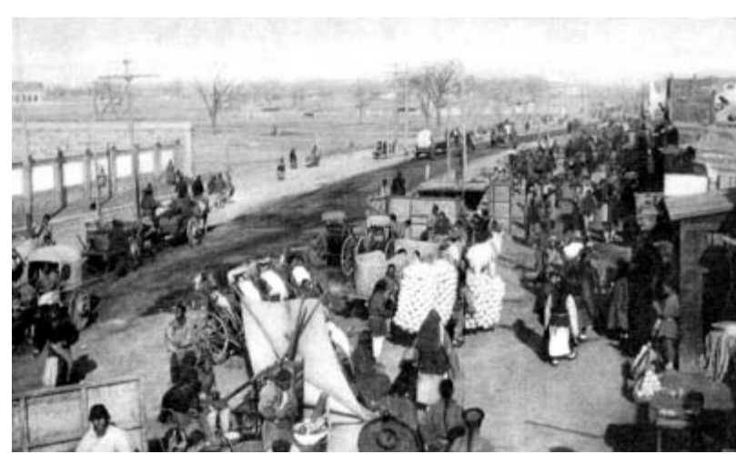
HATAMEN STREET BEFORE MACADAMIZING
